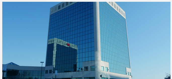
This 10-floor 140,000 sq. ft. office building is monitored 24/7 for leaks and floods by Alert Labs sensors and Insights Platform
