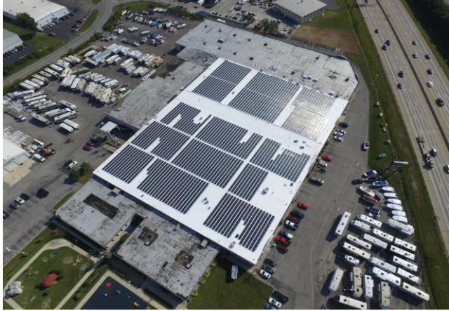
726 kW Rooftop Solar Array Marine Center of Indiana, Indianapolis, IN Design / Build / Transfer
