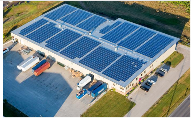
643 kW Rooftop Solar Array Seating Technologies, Goshen, Indiana Feed-In-Tariff
