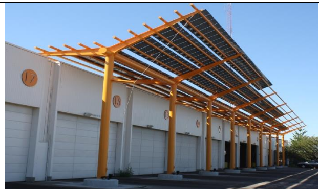
256 kW Canopy and Rooftop Solar Array Toledo Area Regional Transit, Toledo, Ohio Design / Build / Transfer
