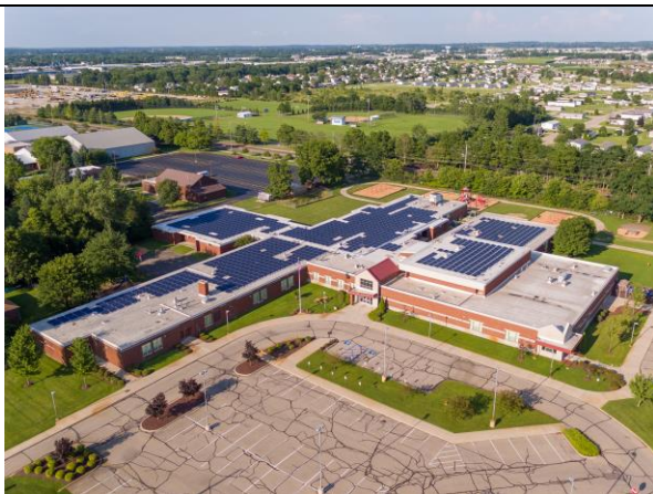
305 kW Rooftop Array Waterford Elementary School, Goshen, Indiana Feed-In-Tariff
