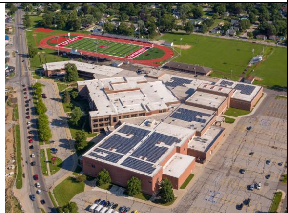
323 kW rooftop Solar Array Goshen High School, Goshen, Indiana Feed-In-Tariff
