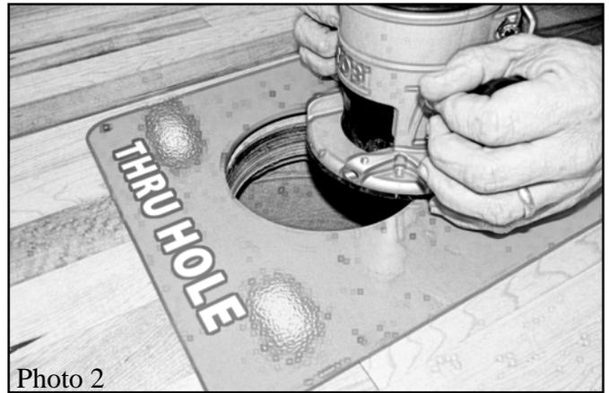
4. Check to insure that the “thru hole” is directly over the center of the existing excavation in the concrete subfloor. If necessary, it is possible to adjust the location as much as 1/2” in any direction without negatively effecting the *Chrome Floor Plate (B)* installation.
