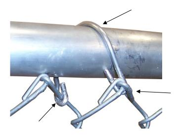
Attach rail tie around two legs of the chain link wrapping tightly around support pipe.
