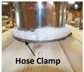
14. Insert ceramic wool insulation around the chimney to provide a protective barrier between it and the wood. Use the hose clamp to secure the insulation around the chimney.
