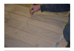
10. On the exterior of the sauna, find the pilot hole. Using a string and pencil, draw an 12" circle on the wood using the pilot hole as the center point.
