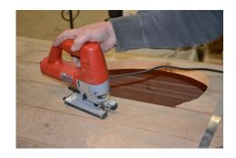
11. Using a jig saw, cut a hole following the line you drew in Step 10.
