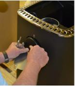
4. The chimney should vent out the top of the sauna. Remove the cover from the top vent hole. Unscrew the hinged plate on the back of the heater and reposition the cover over the back vent hole. Screw the hinged plate back into position.
