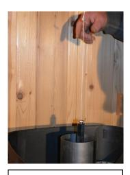
8. Using a plumb line, find the center of the heater flue and mark the corresponding center point on the ceiling of the sauna.
