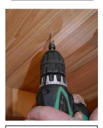
9. Drill a 1/8" pilot hole at the center point all the way through the wood.
