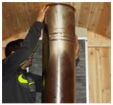
13 . Fit the second chimney section down into the hole and attach to the first chimney section. Rotate to lock into place. Use the wall support bracket to secure the chimney in place.
