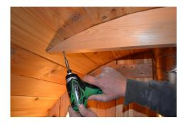
15. Screw the front trim frame piece into place. The distance at which it is positioned from the back wall should be about the same as the width of the depth. Make sure it is level before inserting screws, one on each end of the board into the ceiling of the sauna.
