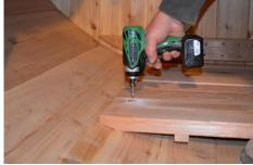
2. Screw the duckboard to the floor using 2" screws.
