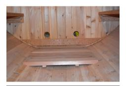
1. Position duckboard base to back of sauna, centering and using a level to insure that the surface is flat.
