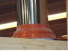
18. Cut the provided boot to the appropriate size so that it forms a tight seal. Position the boot over the heat shield and fasten it into place. Finally, position the cap on the chimney and rotate to lock into place.
