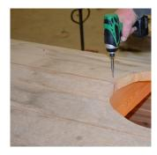
16. From the outside of the sauna, drive screws into the front trim frame piece securing it to the staves.
