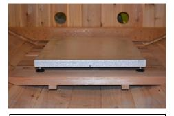
3. Position the protective metal base on the duckboard. Center and allow a gap of 4" from back wall of sauna.
