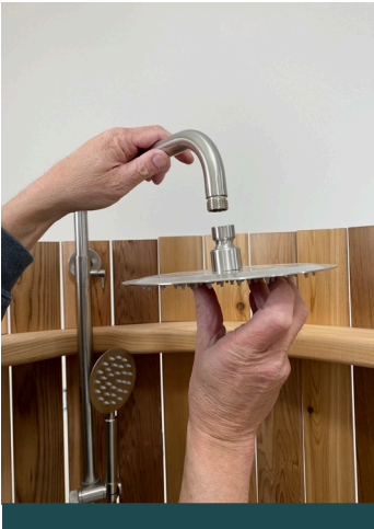
13. Twist the shower head onto the end of the shower stem.
