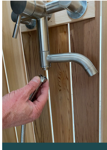
14. Connect the wand to the hose and the hose to the base of the faucet fixture.
