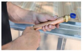
Wrap 3 layers of thread tape around the threads on both ends of the other 2 long pipes.
