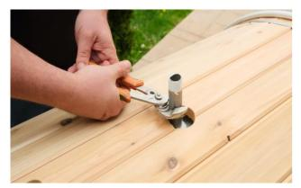
Thread one of the long pieces of pipe into one of the holes on the side of the tub.
