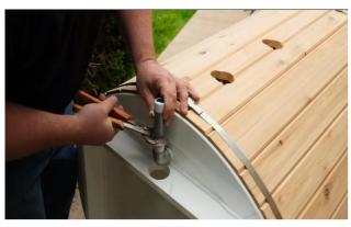
Thread the long piece of pipe into the elbow.
