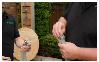
Insert rubber washers into each end of the chiller hoses.
