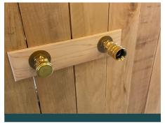
18. The other outlet comes capped from the factory. (If you wish to have your plumber run hot and cold water to the shower, then he will remove the cap, swivel, and adaptor fittings so that he can connect to the ½" water lines.)
