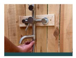
16. Wrap threads of hand wand clockwise with sealing tape and attach wand hose and tighten with wrench.
