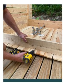
Screw the shelf in place with 2" screws through pre-drilled holes. The shelves will bring stability to the structure.
