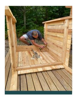
Screw the shelf in place with 2" screws through pre-drilled holes. Be sure the side walls are tight to the shelf before installing screws. The shelves give stability to the shower.
