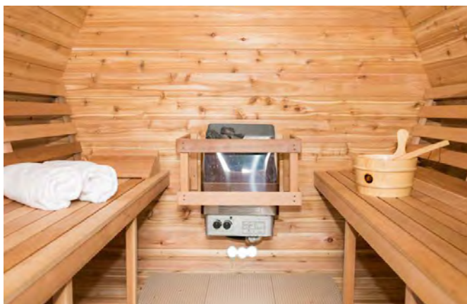
Inlet under electric heater on Back wall
