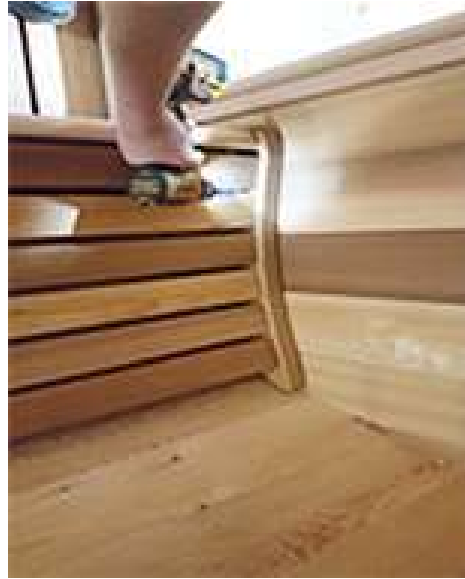
Screw the enclosures and the seat benches to the front wall with 2 ½" (64mm) screws. Screw between the slats to ensure screws are less visible
