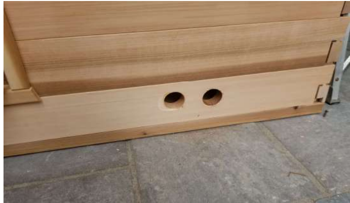
* A 2" diameter hole saw was used in pictures but more holes with a smaller drill size will also work)
