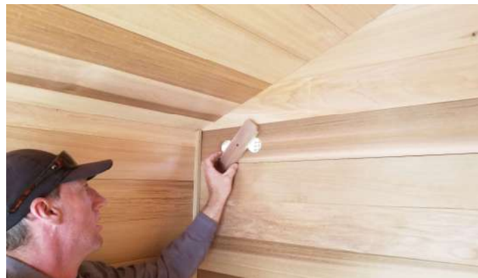
Install the cedar vent cover over the outlet holes on the inside of the sauna with a 1 1/2" screw.
