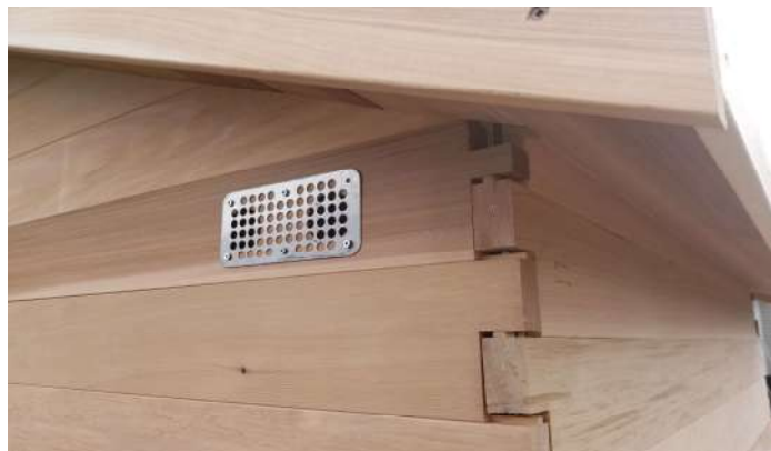
Install the other Stainless Vent cover over the outlet holes on the outside using 1-1/2" stainless steel screws. (6pcs)
