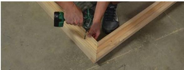
**Note:** Making sure the support frame is square is important for the proper assembly of the remainder of the sauna. You want to make sure this setup phase is done correctly.
