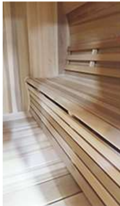
To install the signature back rest, position on wall at desired height and fasten with 2 1/2" (64mm) screws.
