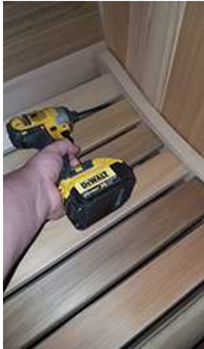
Screw the seats in place using the same method as in previous step.
