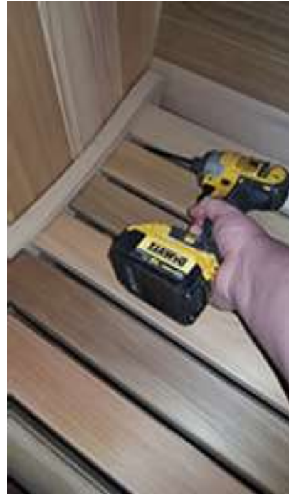
4 screws in each seat, 2 in front and 2 in the back. Screw between the seat boards to make the screws less visible.
