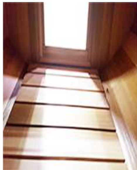
Ensure the flat floor is centered in sauna and that it is level, you can use the door frame to confirm it is level.
