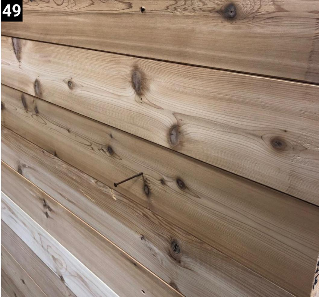
Screw 3" screws into all remaining pilot holes on the side walls.
