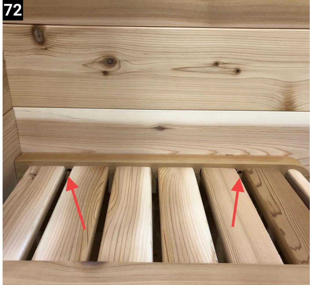
72 Secure porch bench to front wall using 2" screws into the pilot holes between the slats
