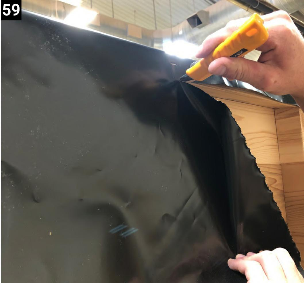
Once secured, cut roof membrane to the edge of the roof boards
