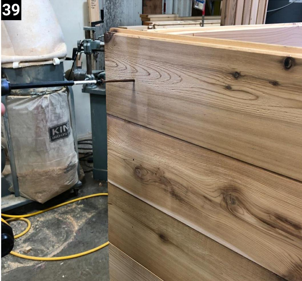
Then attach to the front and back wall with 3" screws.
