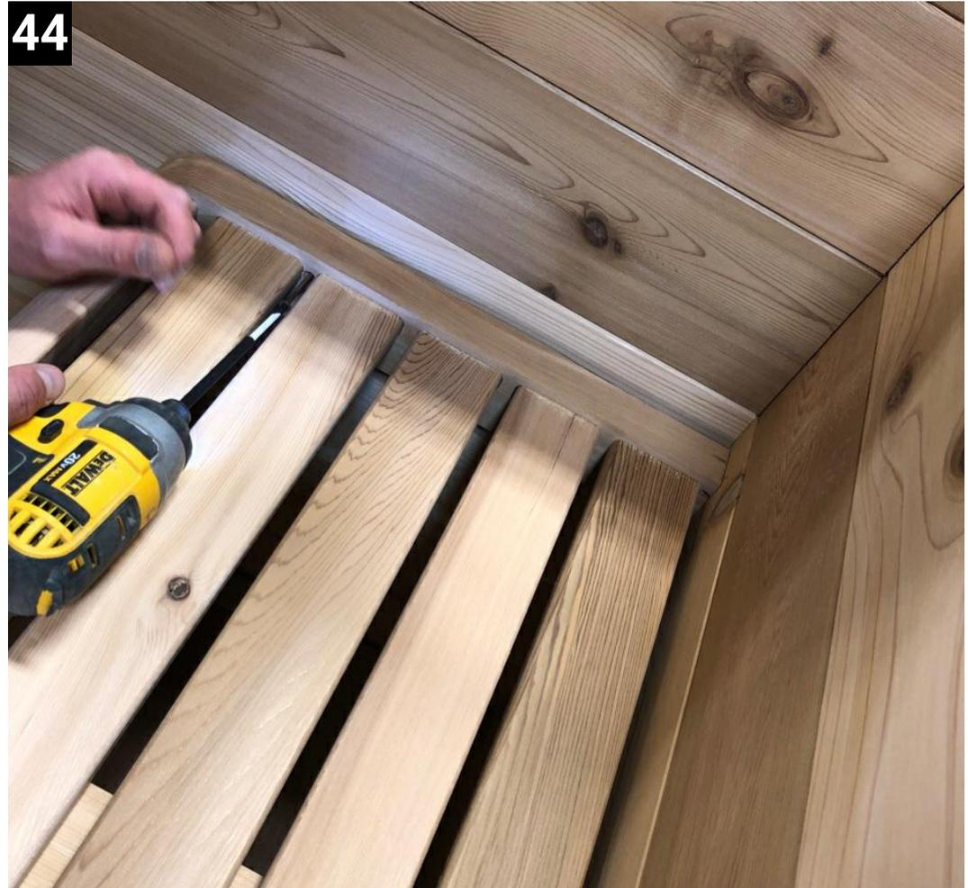
44 Attach top bench to the wall with three 2" screws in each side.
