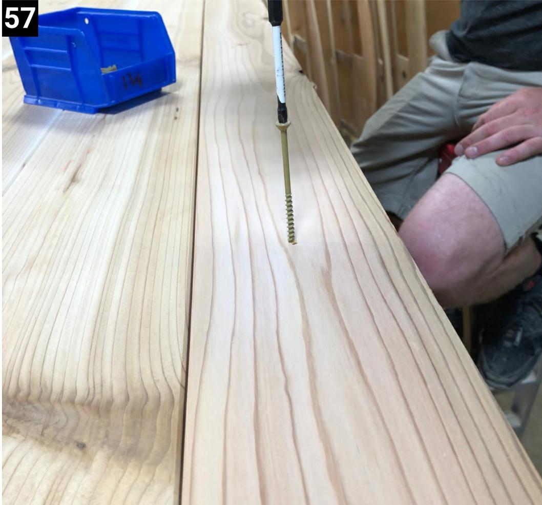
Secure the roof to the front and back wall with three 3" screws in each
