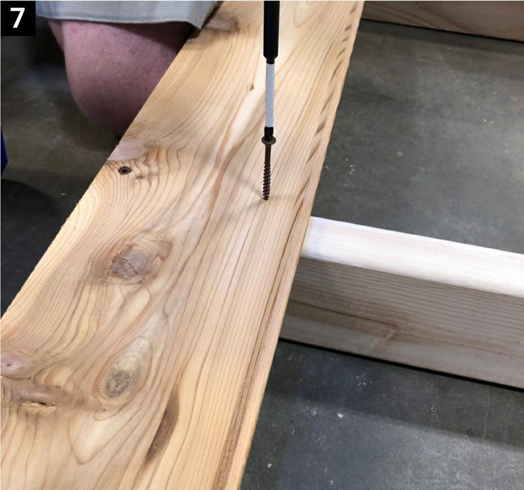
7 Sink two 1 3/4" screws into each 2x4 except for the center 2x4, leave it with no screws. No hot screws on bare feet.
