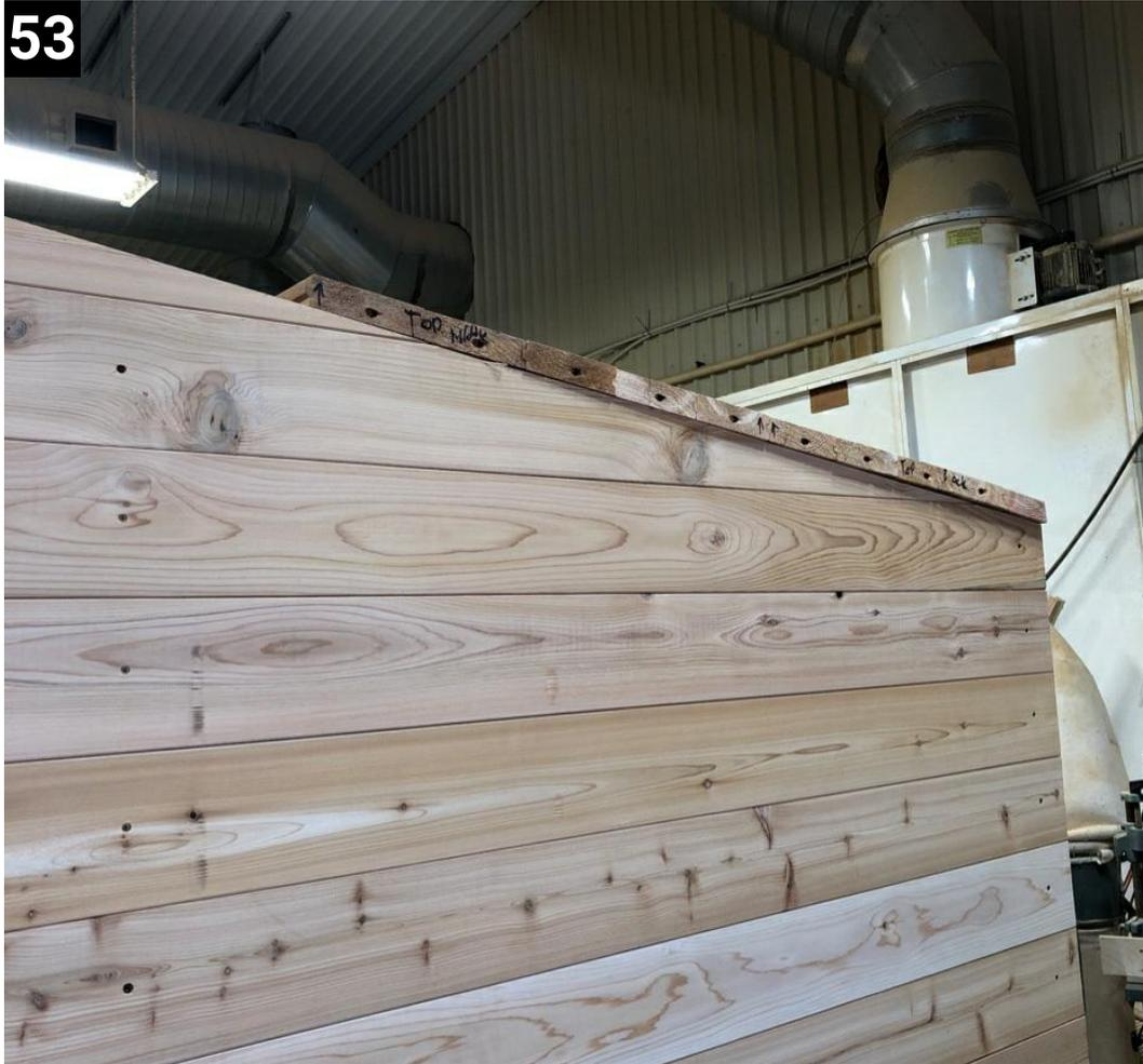
Place top middle piece on the roof and attach it to the top back piece with 4" screws
