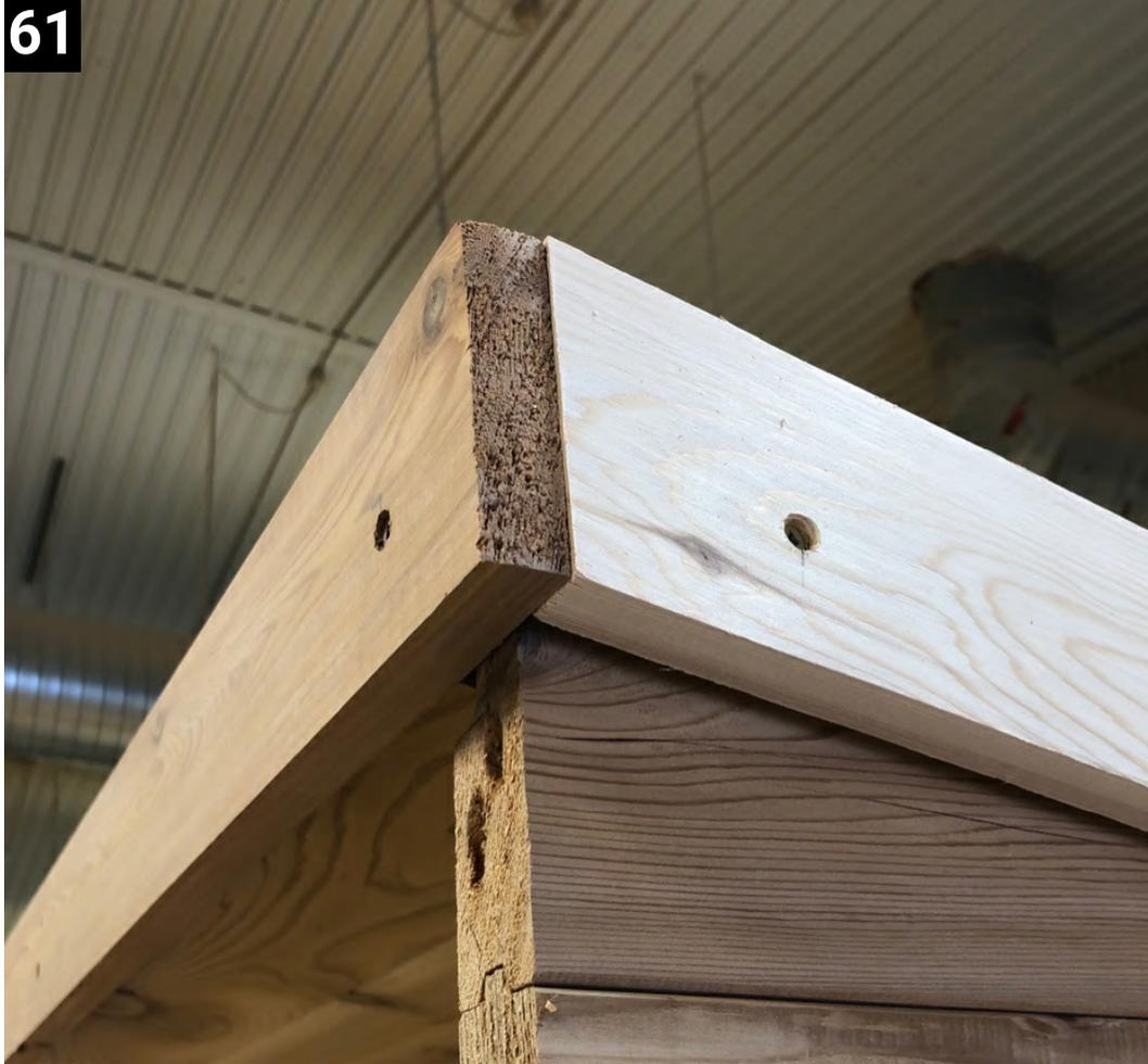
61 Install side pieces with the 10°mitre on them flush to the front barge board.
