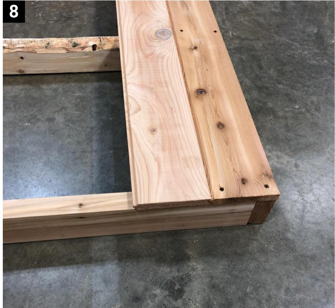
8 Place down second board and make sure it is flush to the edge of the first board.
