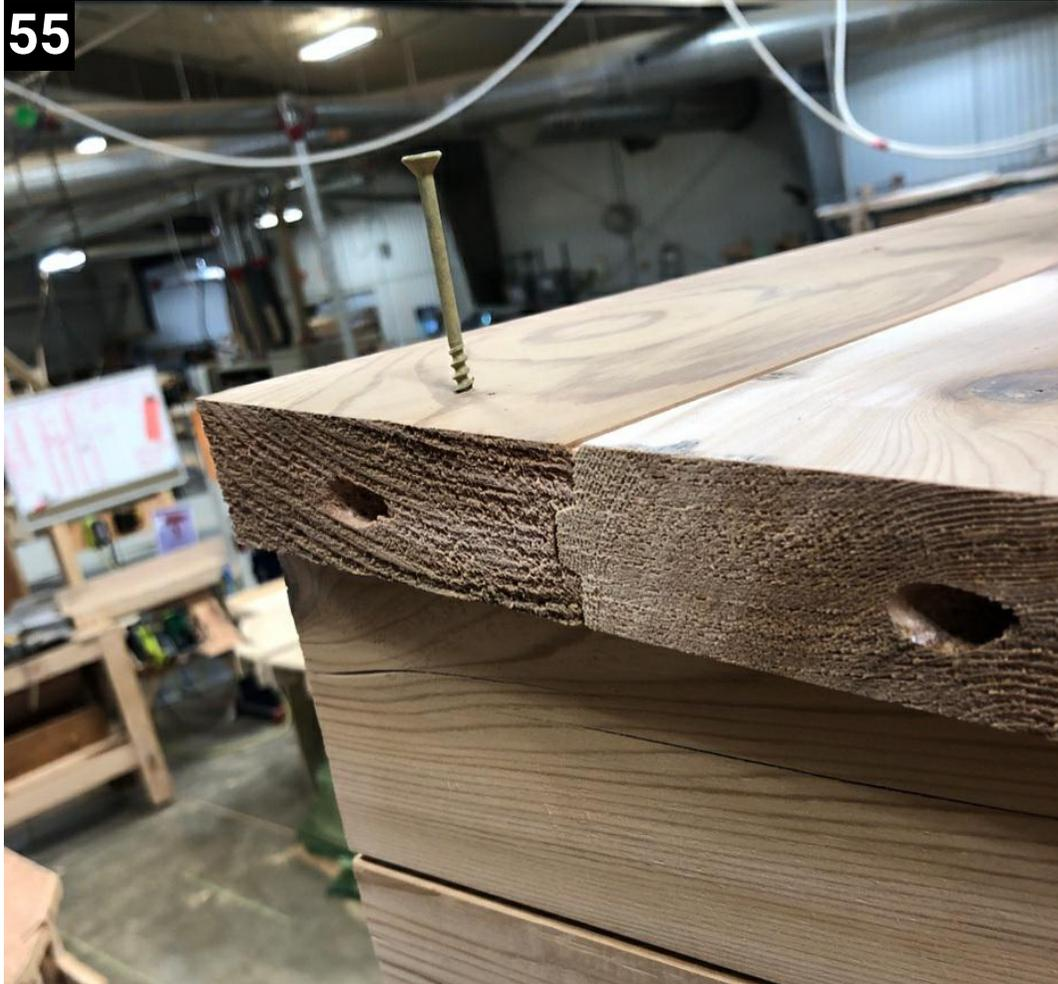
Center the roof on the body of the sauna and secure down with 3" screws
