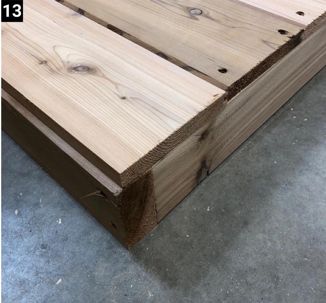
Use the other piece with a flat edge as the last board of the floor. Attach the same way as the rest
