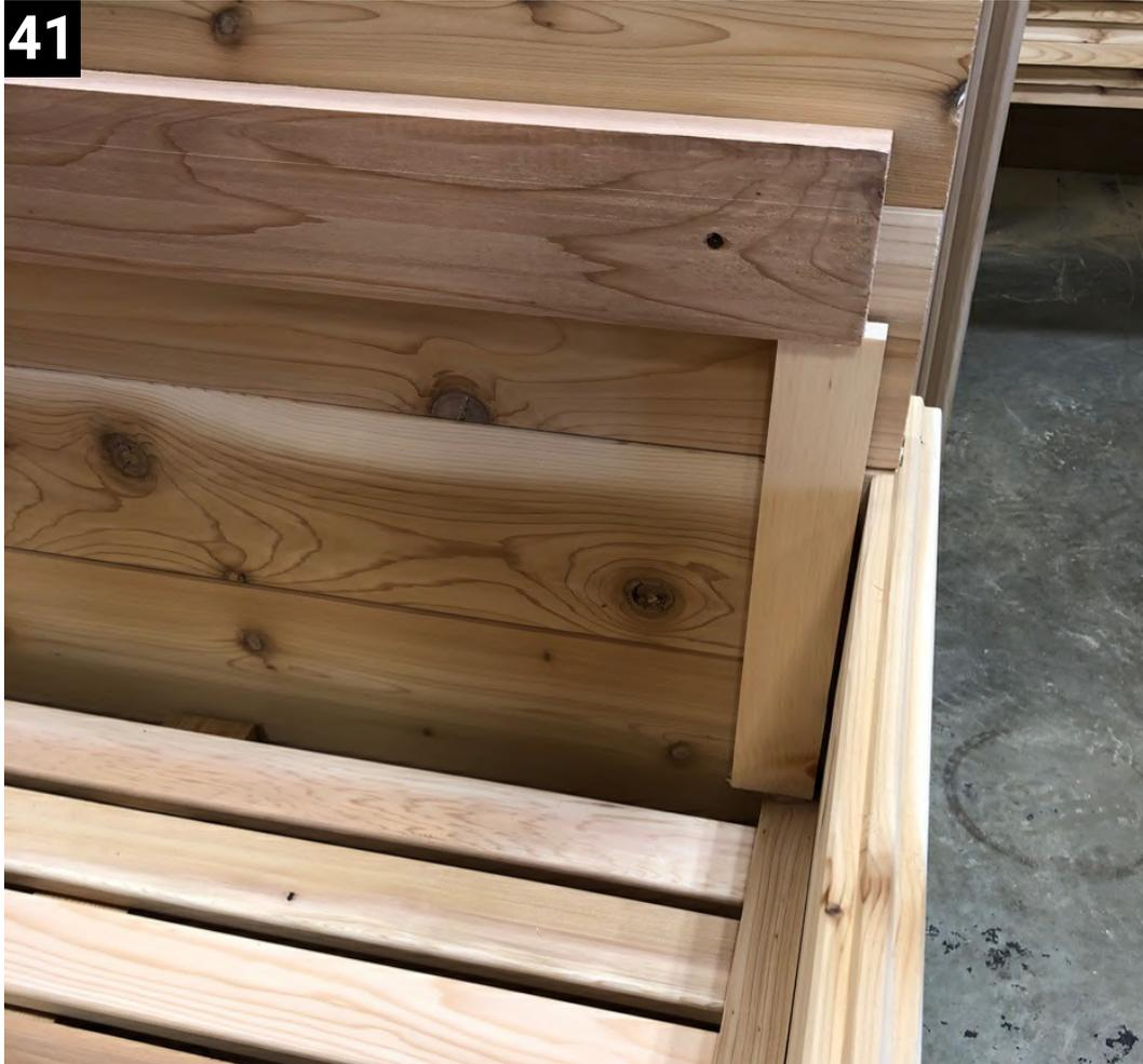
41 Place the bench support 2x4 on top of the bench spacer and screw to the back wall with five 2" screws.
