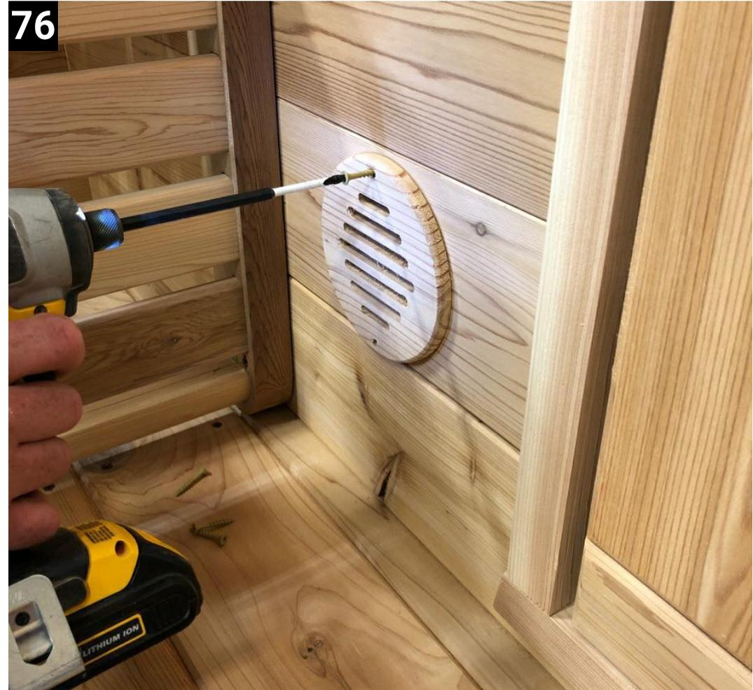
76 Put vents into the outside holes. Use 1 1/4" screws
