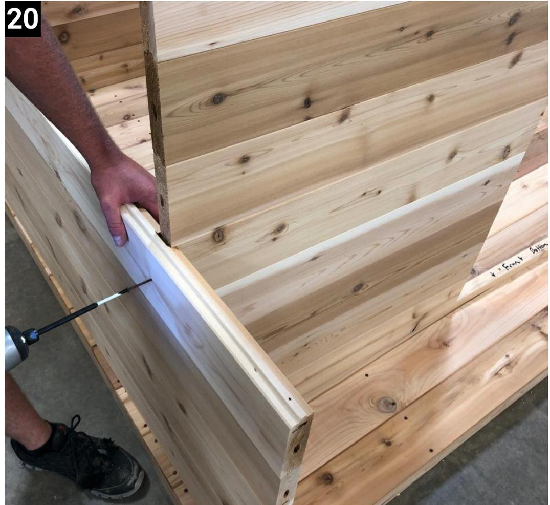
Slot the side that was just attached into the side wall. And attach using 3" screws.
