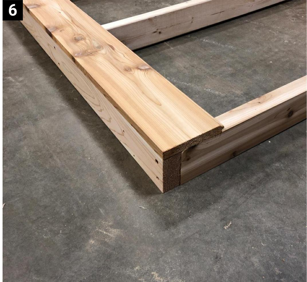
Start the floor boards off with one that has a flat edge. Align the edge flush with the front and corner of the floor frame.
