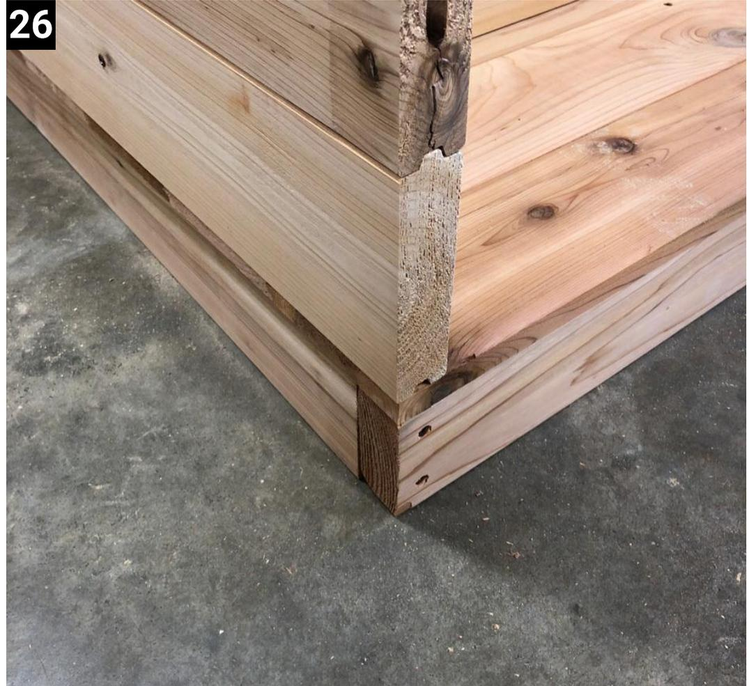
Flush up the front of the walls to the front of the floor frame, and center the sauna on the floor.
