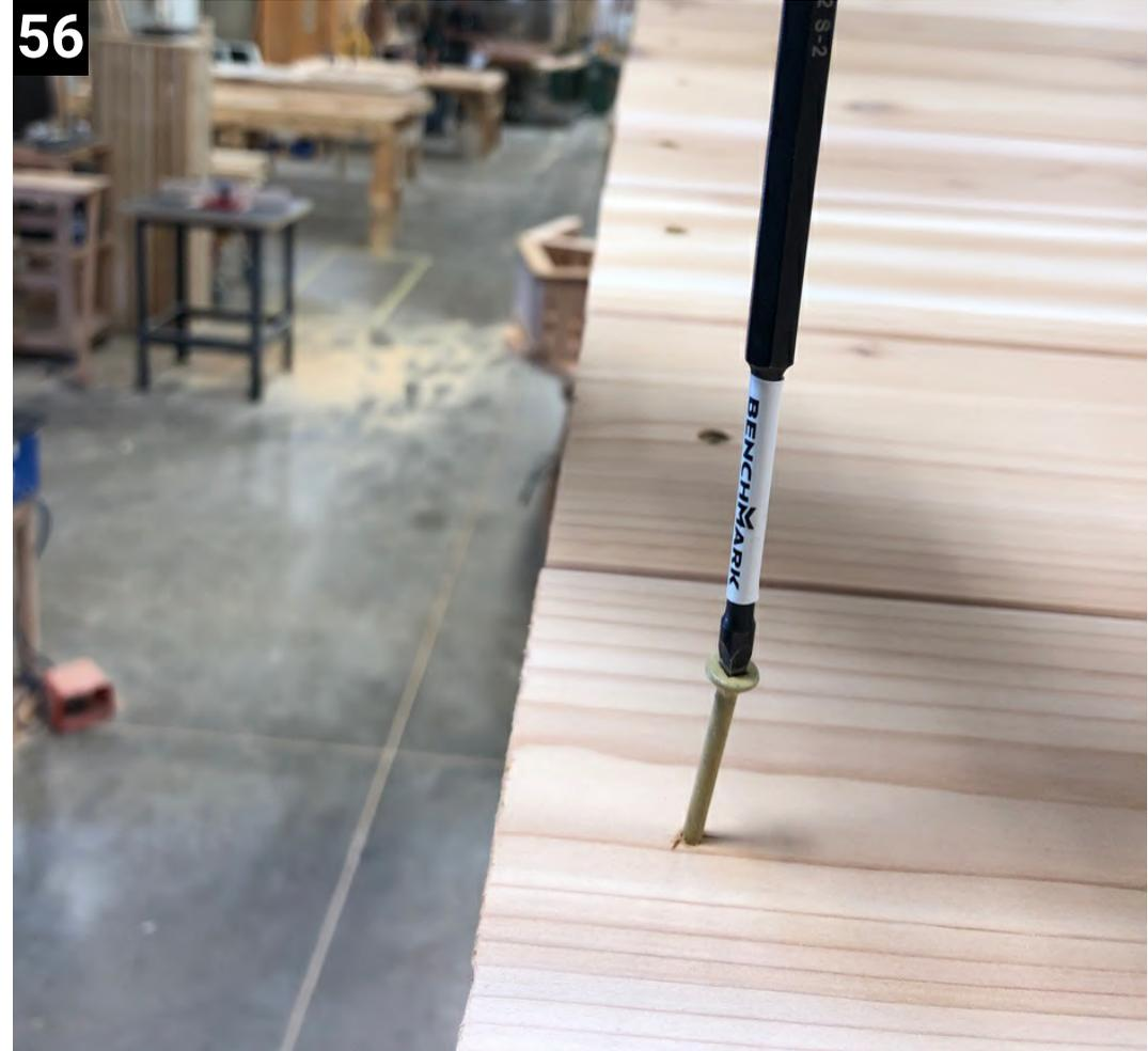
Sink a 3" screw in each end of every roof board.
