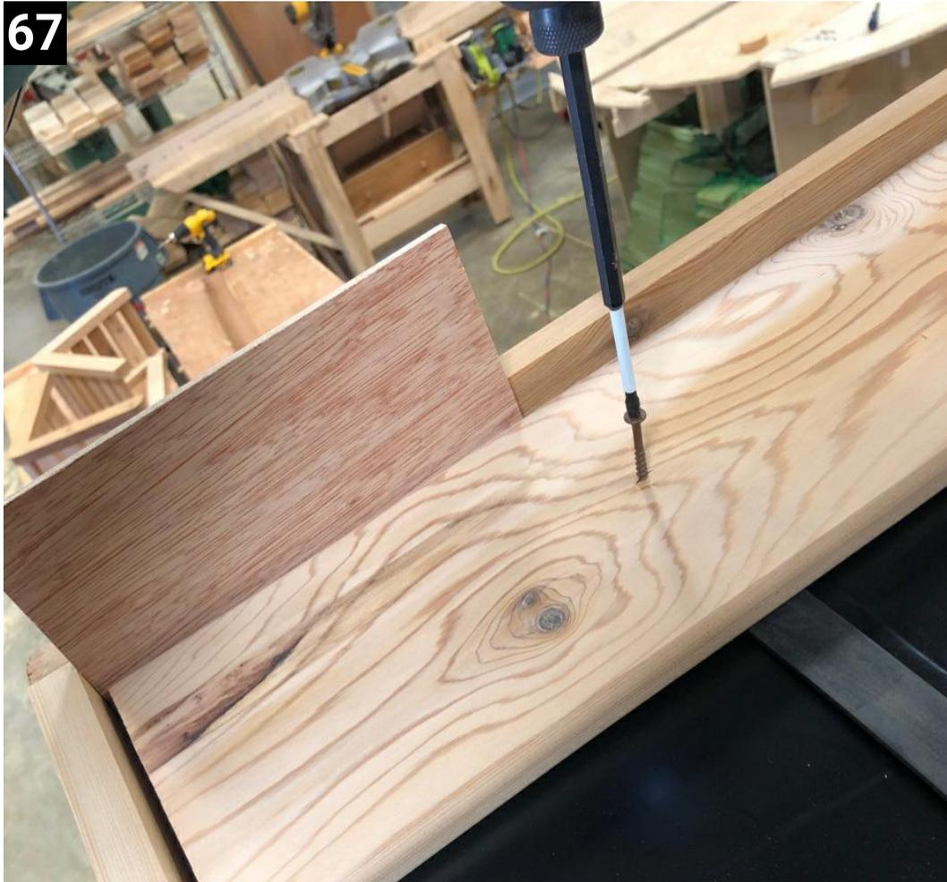
67 Space the first roof board with the plywood away from the front barge board. Use a 1 3/4" screw to secure it. Make sure to drive the screw through the neoprene strip
