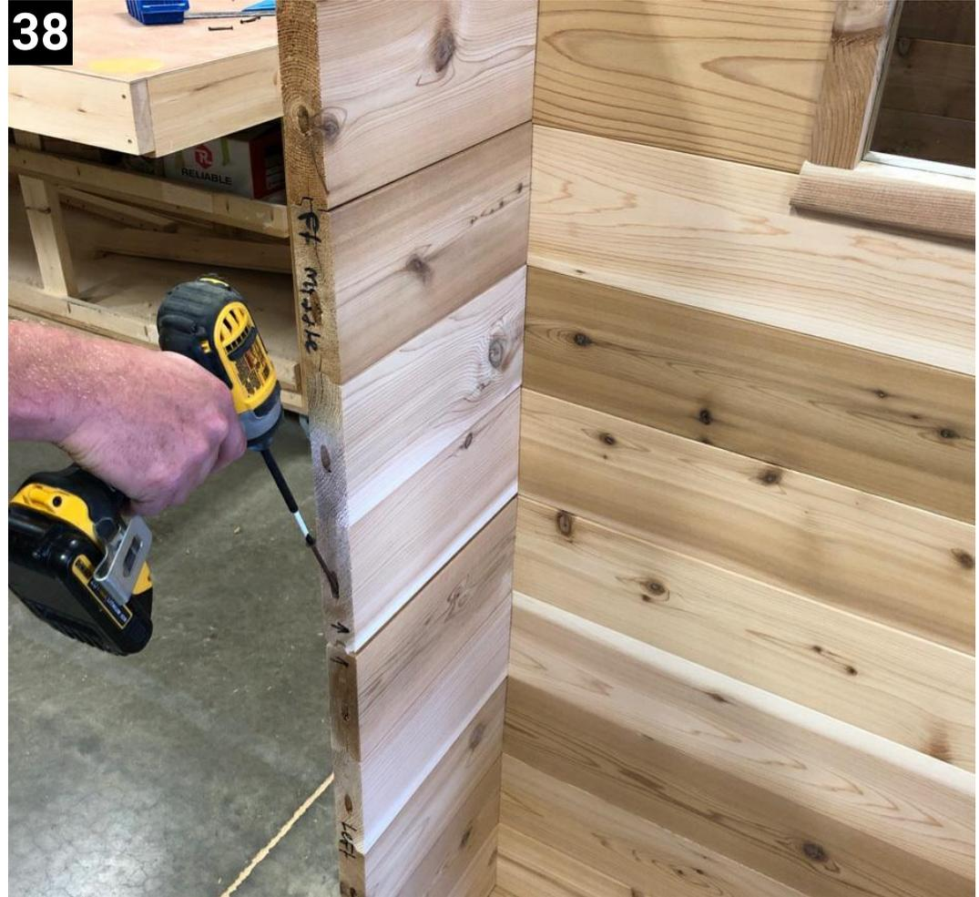
Slot in the middle of each side wall and attach to the bottom with 4" screws
