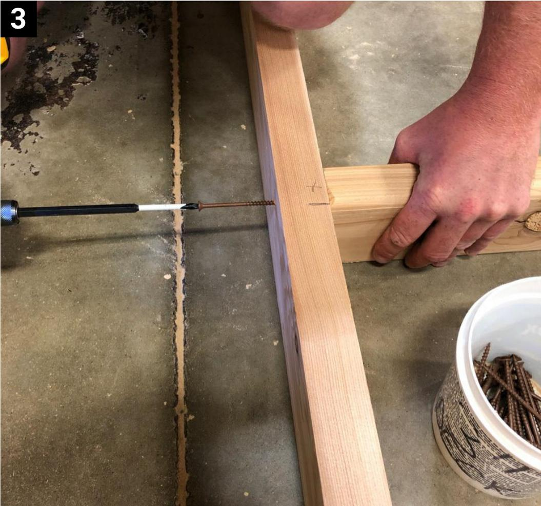
3 Attach the 67" 2x4s with 3" screws. Line up all boards on the previously marked spots.
