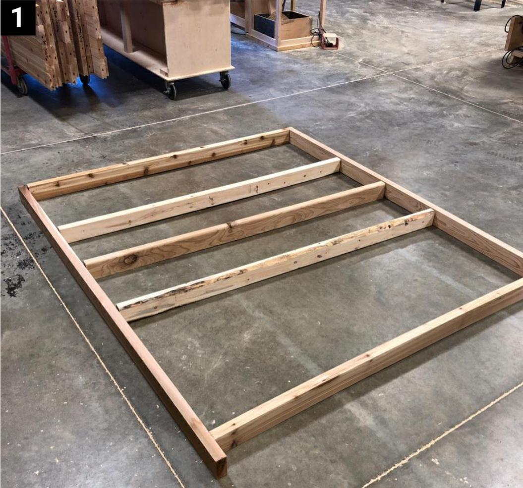
Start the assembly on a nice firm level surface. Start the floor by laying out the two 82 3/4" 2x4s and the five 67" 2x4s.
