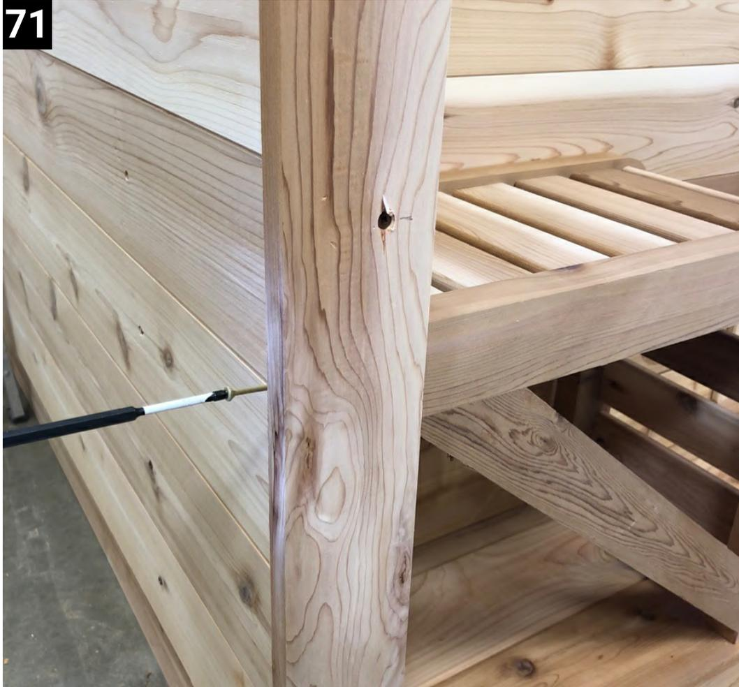
71 Secure the porch bench through the wall with a 3" screw into the bench arm.
