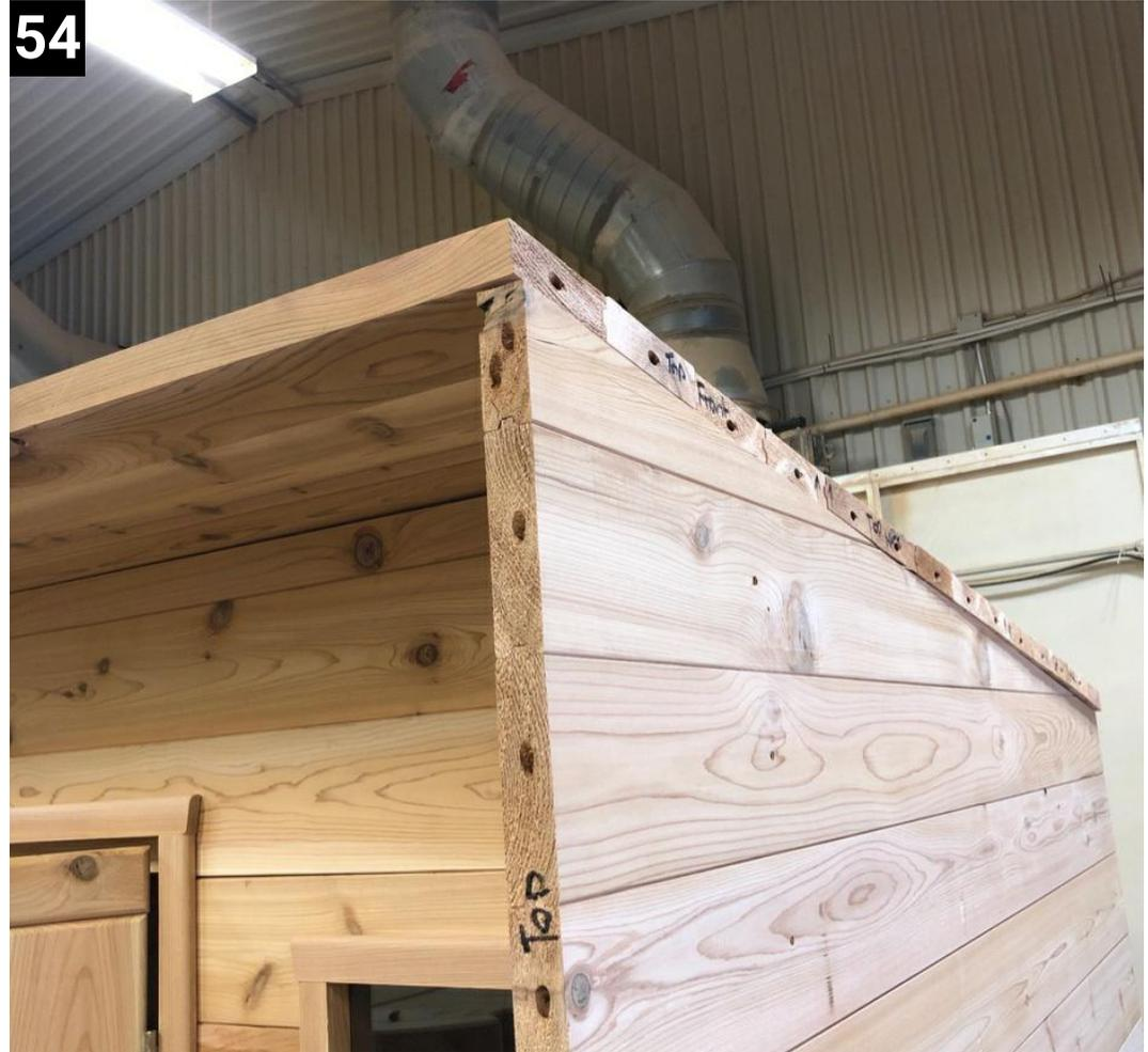
Place the top front piece on, and screw to the top middle piece with 4" screws. Make sure arrows are pointing up
