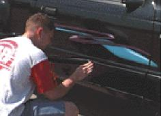
5. A roll down with a hard rubber hand roller is recommended to assure complete wet-out of the adhesive to the vehicle surface. Apply firm pressure while rolling the moulding to properly wet-out the adhesive.
