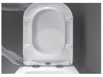
Aim at the holes and adjust the hinge base to make the seat cover and pan match.
