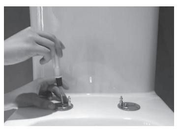
Tighten the setscrew but not to the end in order to adjust the seat cover properly.
