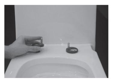
Insert the screw on the hinge base into the holes on the pan.
