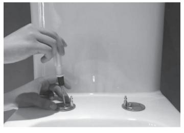
Lock the support completely on the ceramics and cover with stainless steel cover.
