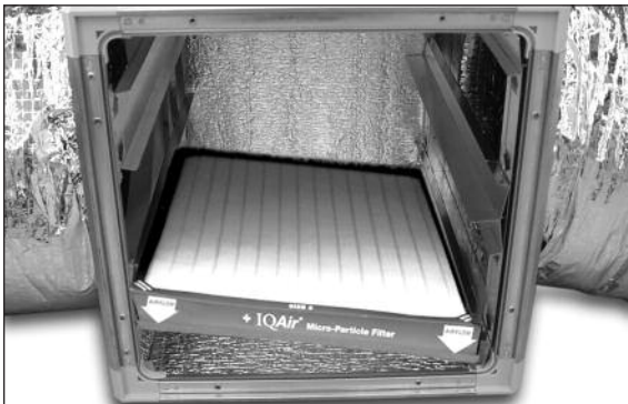
5. Insert new filters starting from the bottom.
