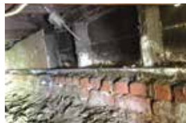
FLOOR-TO-WALL CONNECTION AT PARALLEL JOISTS
