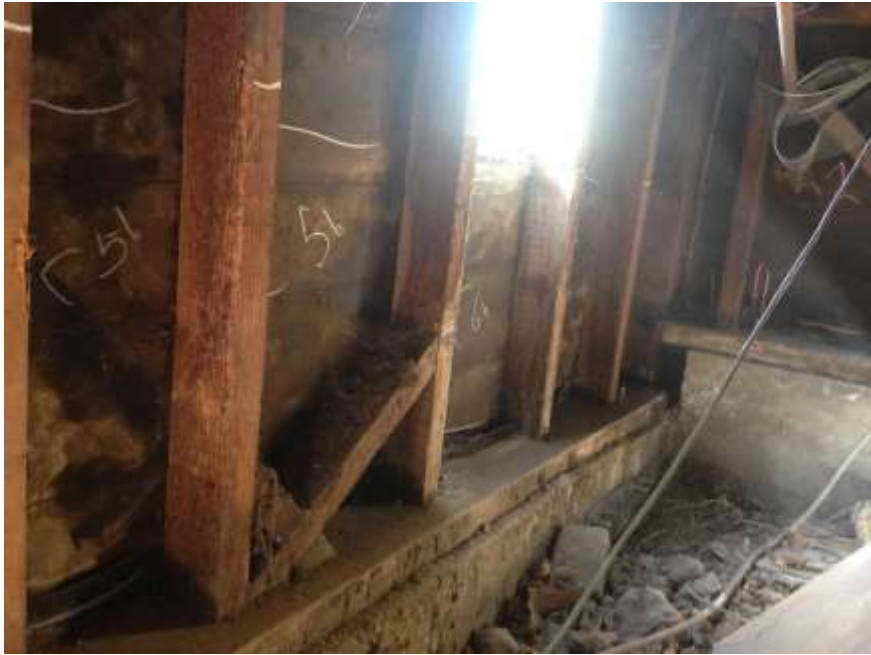
Crawlspace wall before
