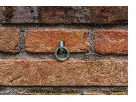
Option A. tested fixing eye in masonry
