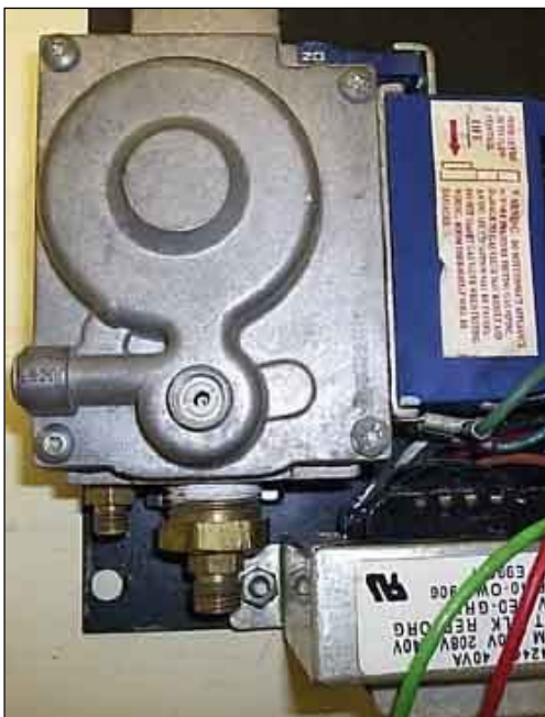
Photo 13. Inside view, adjustment screw.
