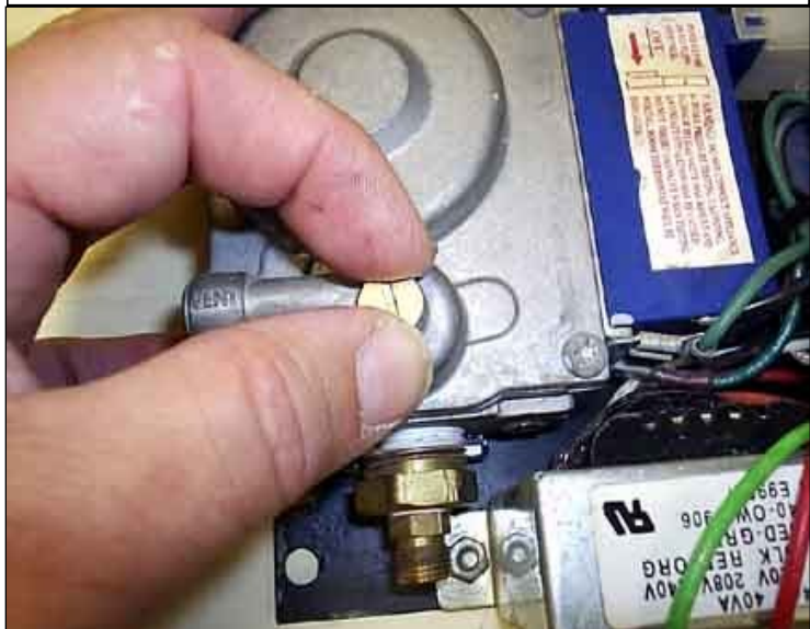
Photo 14. Adjusting valve adjusting screw
