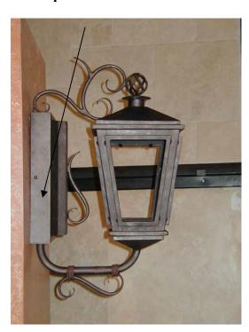
3. Using a crescent wrench, disconnect the incoming flex hose from the top connection on the units gas valve.
