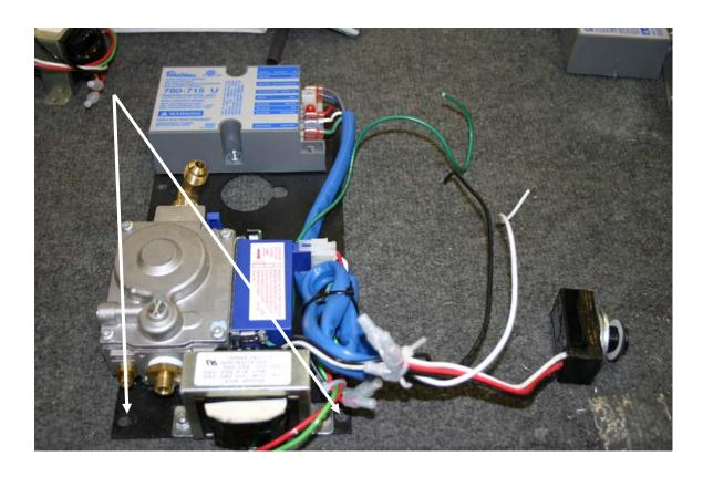
7. Reverse the steps to install the unit. Check to make sure the inner gas on/off switch is in the on position. The picture shows the off position. Turn switch to the on position if necessary.
