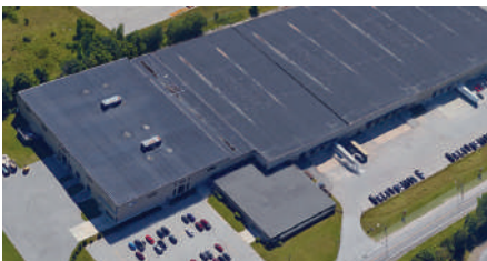
Barrie, ON (CAN) - High Performance Doors
