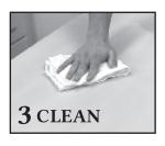
If you're applying the Epoxy Resin over an existing Giani® Topcoat, then thoroughly clean the finish with mild dish soap and water. Do NOT use any other cleaners. If you're applying the epoxy topcoat over a new mineral or veining application, then there is no need to clean.
