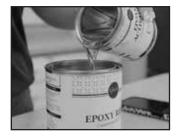
With your safety glasses and gloves on, open the contents of the first set of Epoxy Resin Topcoat. Keep in mind that a set is 1 can of Resin and 1 can of Activator.
