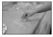
Allow your veins to dry for 2 hours before attempting to repair the section. Once dry, simply use the included #600 grit sandpaper to smooth out the peaks of the veins. Take care not to sand too aggressively. You really just want to level the height of the vein. Once your repair section is smooth, wipe up the sanding dust with a damp cloth and allow the surface to dry.
