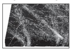
Adding too many veins, spraying too close to the countertop, and holding the nozzle down too long are the most common mistakes while creating veins. However, with a few technique corrections, they are easy to avoid. Just remember to maintain proper distance from your countertops and stick with short, controlled bursts of the Vein Spray. This will keep your application looking natural.
