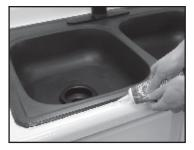
AFTER MIXING THE COMPONENTS, YOU HAVE ABOUT 30 MINUTES TO COMPLETELY COAT THE SECTION before it stops flowing adequately. It takes about 5 to 10 minutes to coat one 6-foot section.
