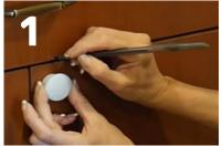
Identify a suitable location to lock. Mark location with pencil where the lock will be installed.
