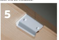
Take off the adhesive cover from the latch and install it flush with the cabinet edge and in the center of the pencil mark.
