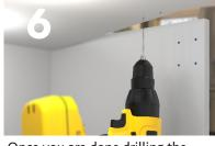
Once you are done drilling the holes for the lock, it's time to drill holes for the latch.
