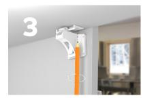
Mark the latch's 2 pilot holes with a pencil.
