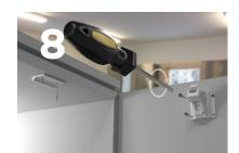
Optionally, remove the stickers from the latch and lock. Screw the lock and latch into place.
