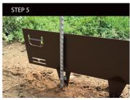
5. Next you need to insert the pin through the top of the clip and start to drive the pin into the ground using a hammer. Take care when hitting the pin head not to make contact with the top of the edging as this may cause damage to the powder coating.
