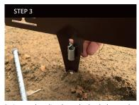
**3.** Insert the clip through the hole on the ground spike. You can have the extension pin on either the front or the back of the edging whichever suits your installation best, however it is easier to insert the clip from the front and have the pin at the back of the edging due to the concaved design of the ground spike.
