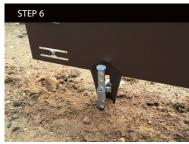
**6.** Once you have installed all the additional extension pins that you require you can tap the edging back down to the desired height using a mallet and a block of wood. This will push the clip to the top of the hole where it becomes slimmer creating an even tighter grip on the ground spike.
