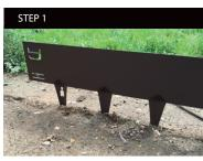
1. If the edging has already been installed, but just isn't quite sturdy enough you can easily add the extension pins for additional support. First you will need to expose the clip hole on the ground spike either by slightly lifting the edging or digging away the surrounding soil.
