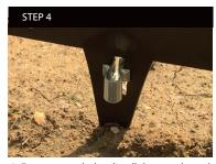
**4.** Ensure to push the clip all the way through until the two smaller flanges are through the hole and lock into place. It may be necessary to squeeze the back of the clip to enable the two flanges through the hole. On the HD edgings it is easier to angle the clip slightly to allow the one flange through at a time.
