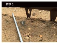
2. On the 1075mm edgings there are 3 available clip holes. On the 2275mm edgings there are a total of 5 holes. It may not be necessary to use an extension pin in each available hole, It will depend on ground conditions.
