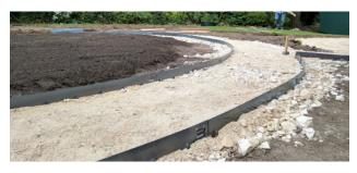
All of our edgings except our weathered steel (Cor-Ten effect) have a 20-micron Galvanised Zinc coating. Our (RAL) coloured edgings have a further 110-micron UV resistant polyester powder coating preventing colour fade, forming a durable scratch resistant barrier guaranteeing a 20yr plus product life.
