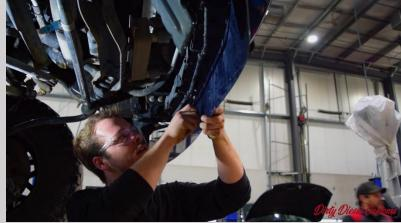
Step Three: With the new valance, start installing the new bolts from the inside out, leaving them slightly loose so you can align all 11
