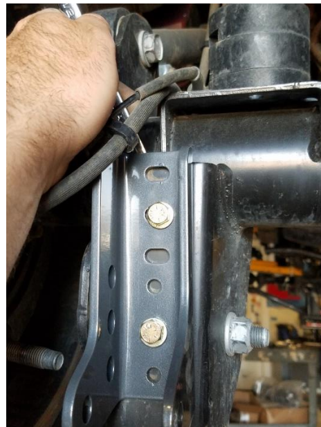
Figure 10. Final Install and Tightening of Fasteners
