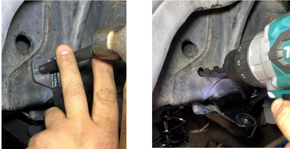
Figure 12 and 13. Center Punched and Drilled Frame Rail (1/2" Drill Bit)
