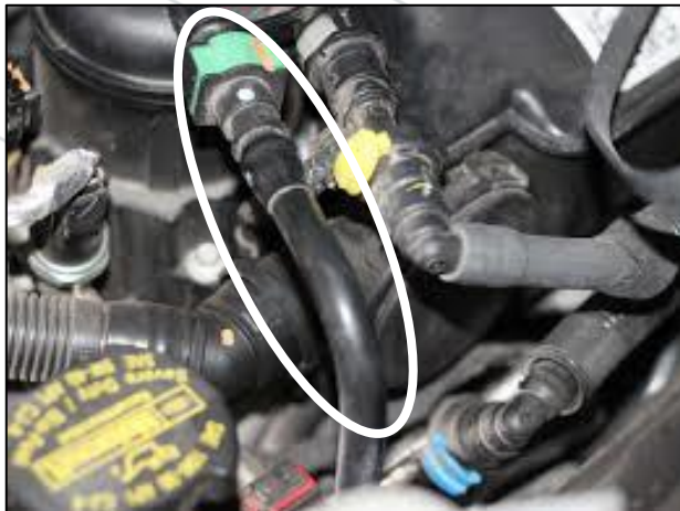
Figure 9: Fuel line is removed and not reused
