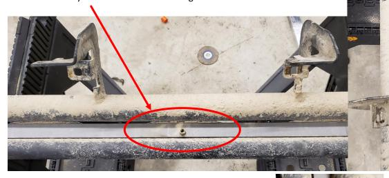
**Step 3:** Use a 1/4" drill bit or a punch to mark holes for drilling.
