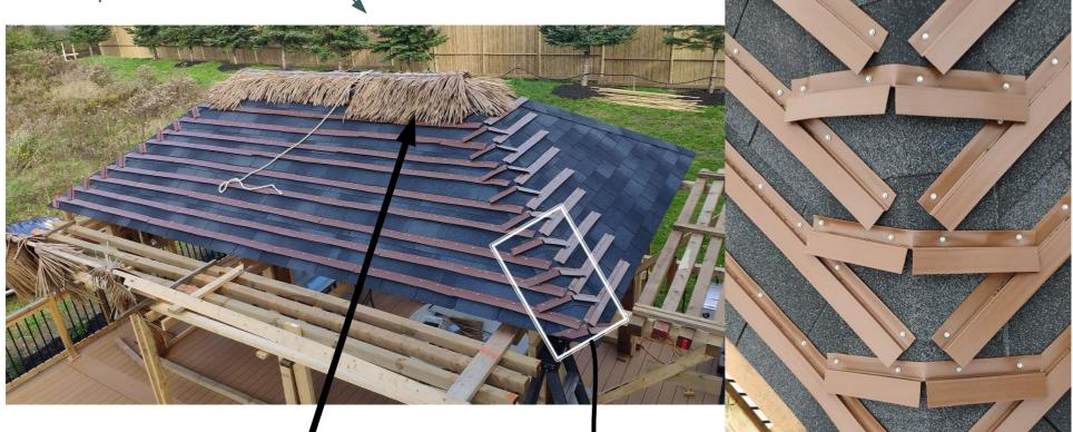
5 Install thatch from top to bottom to provide working surfaces with better traction
