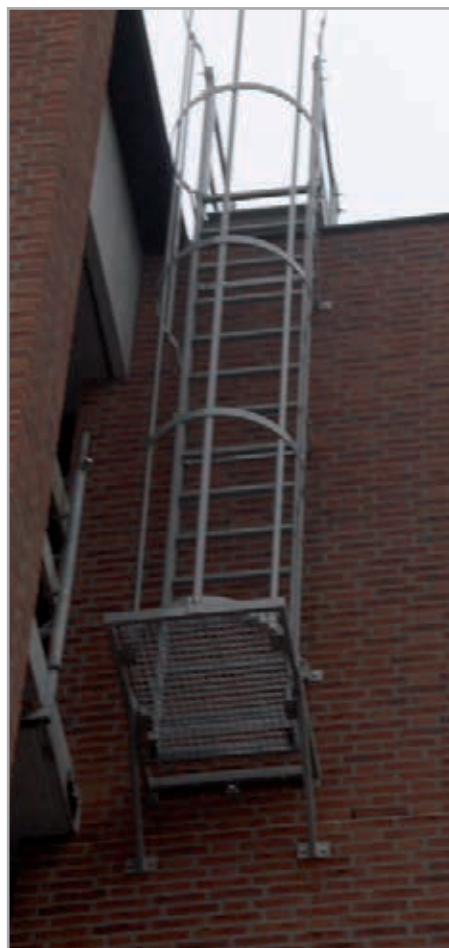
Hoop ladder with access from above and step-off platform for side step-off
