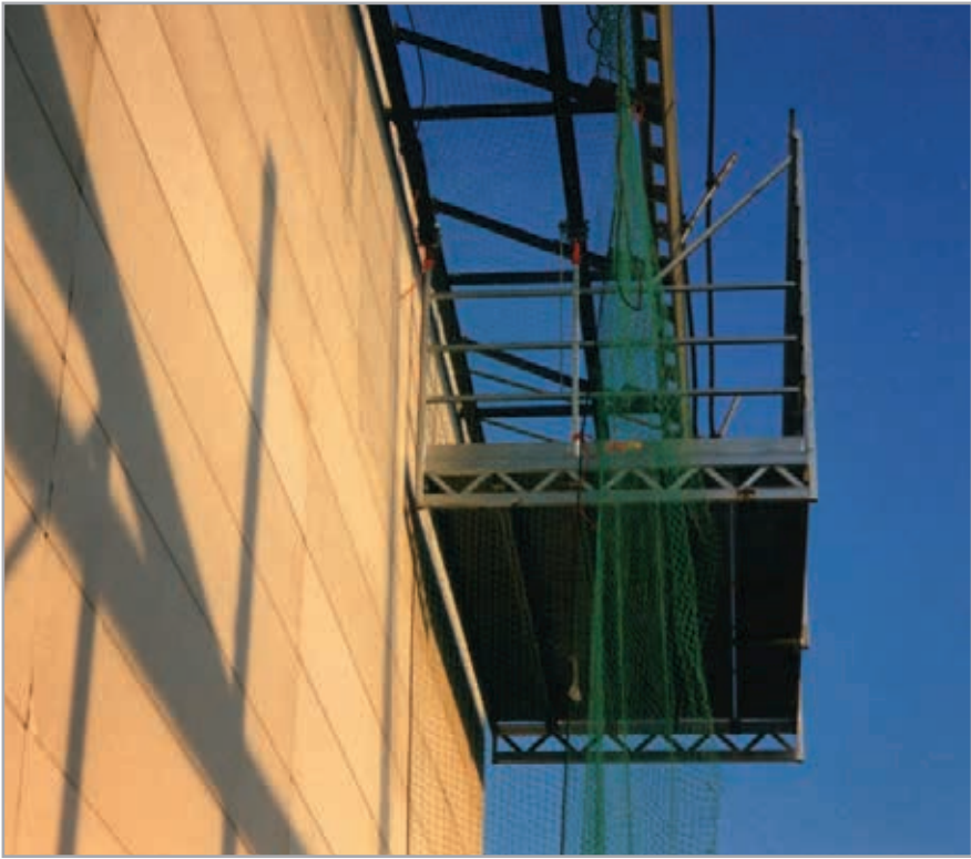
Suspended scaffold with extra wide work floor
