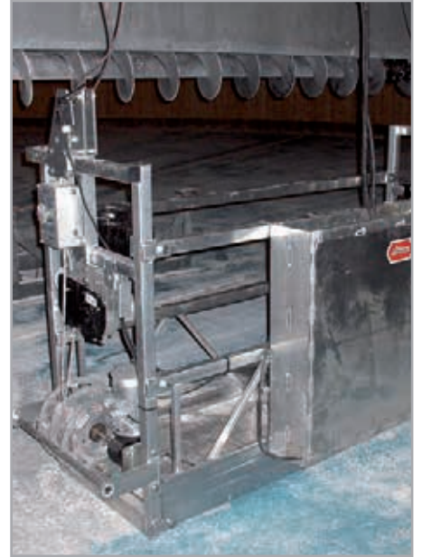
Suspended platform in silo
