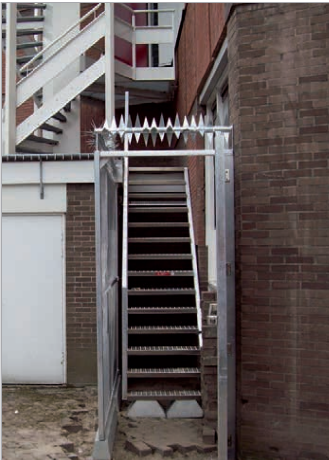
Fire escape stairs with emergency door and anti-theft railing
