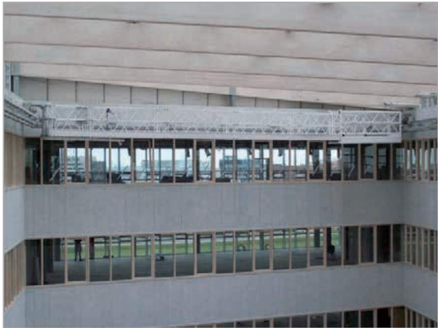
Working platform in building
