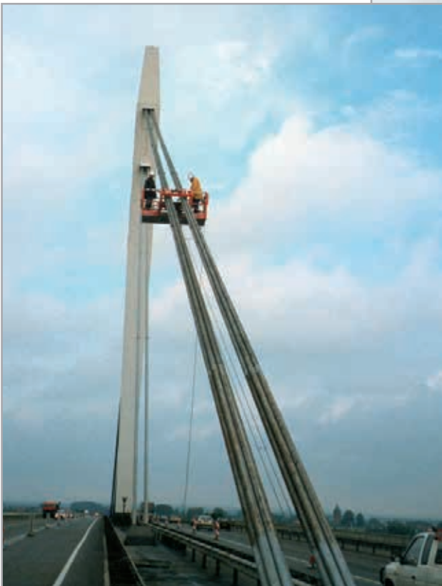
Mobile working platform on the suspension cable of a bridge
