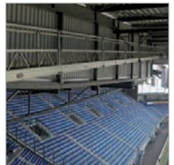
Maintenance platform Football Stadium
