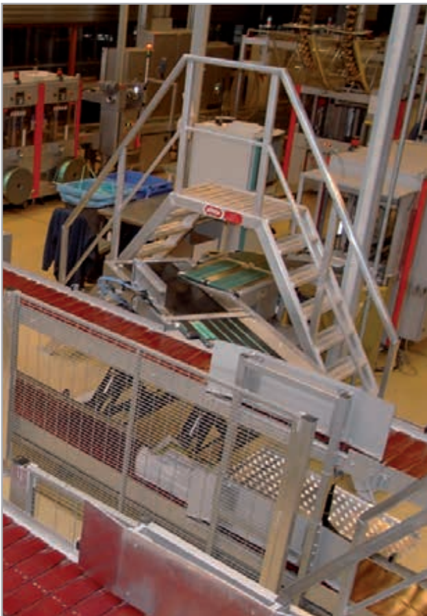
Industrial step-over/stairs for conveyor belt
