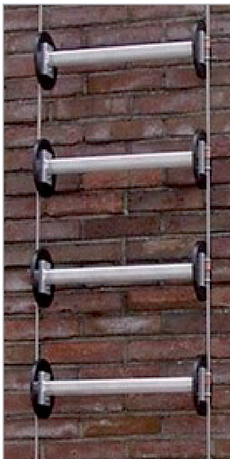
Steel cable ladder rung connection
