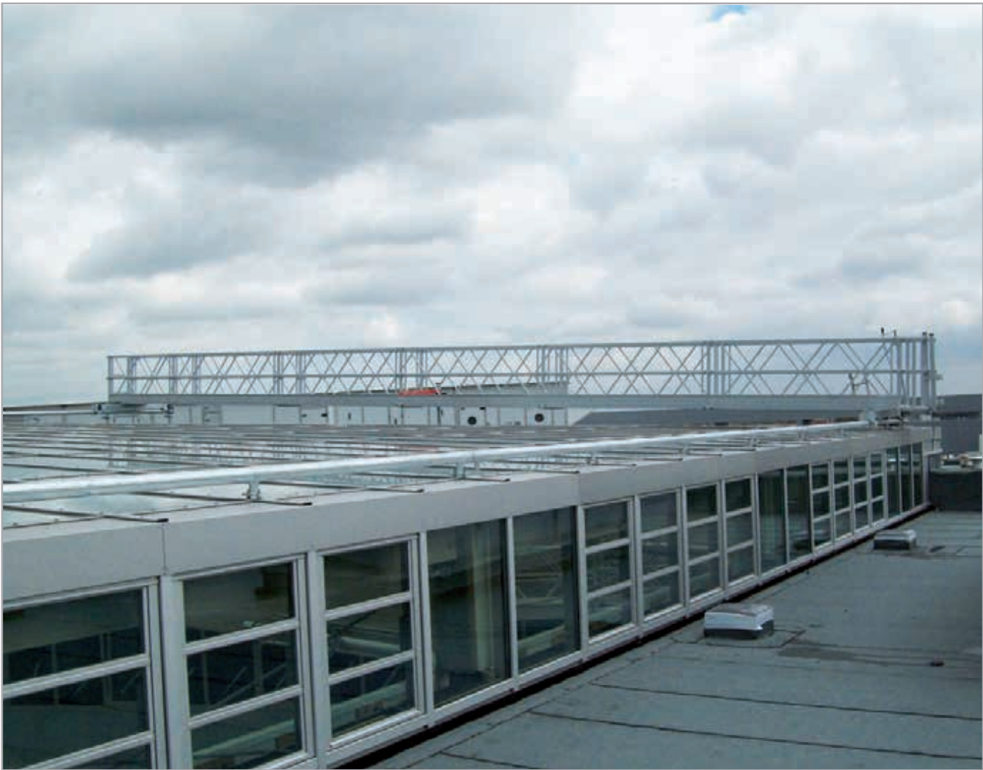
Working platform/walkway over glass roof
