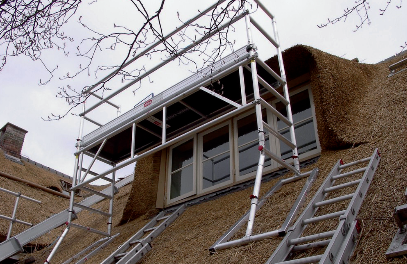
Dormer window scaffold for a straw roof
