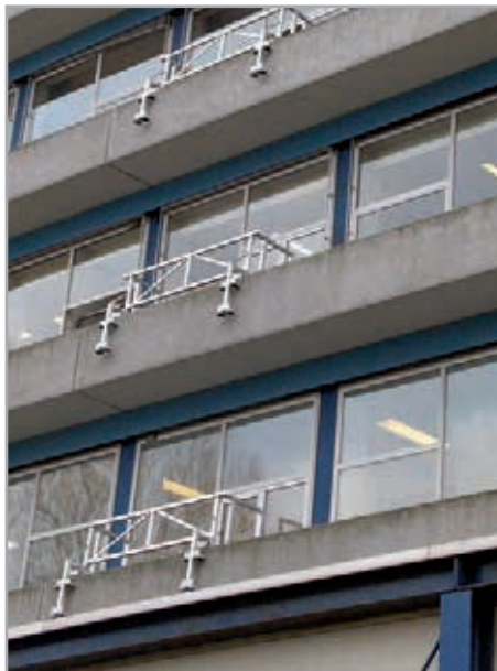
Transportable railings for balconies
