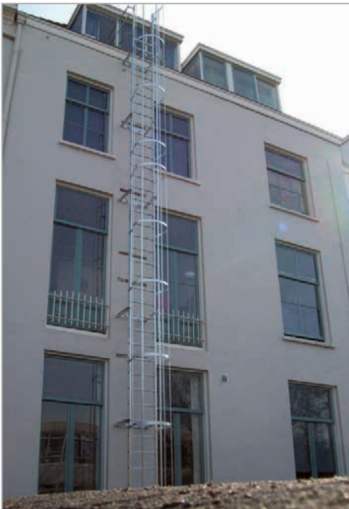
Hoop ladder with extended wall and suspension supports
