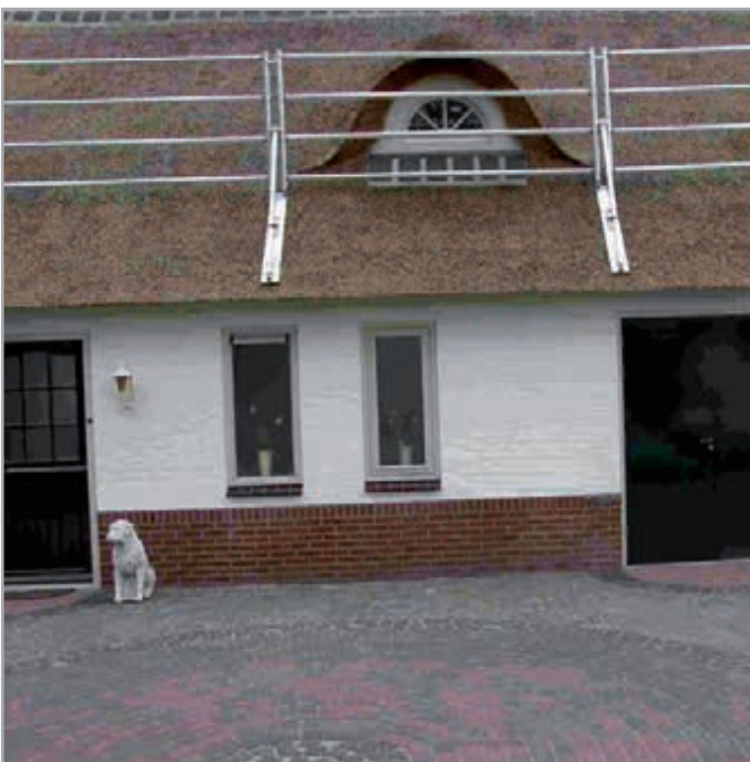
Fall protection for sloping thatched roofs
