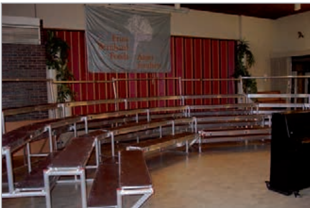
Podium made out of scaffolding components
