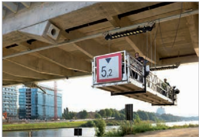
MHB under bridge
