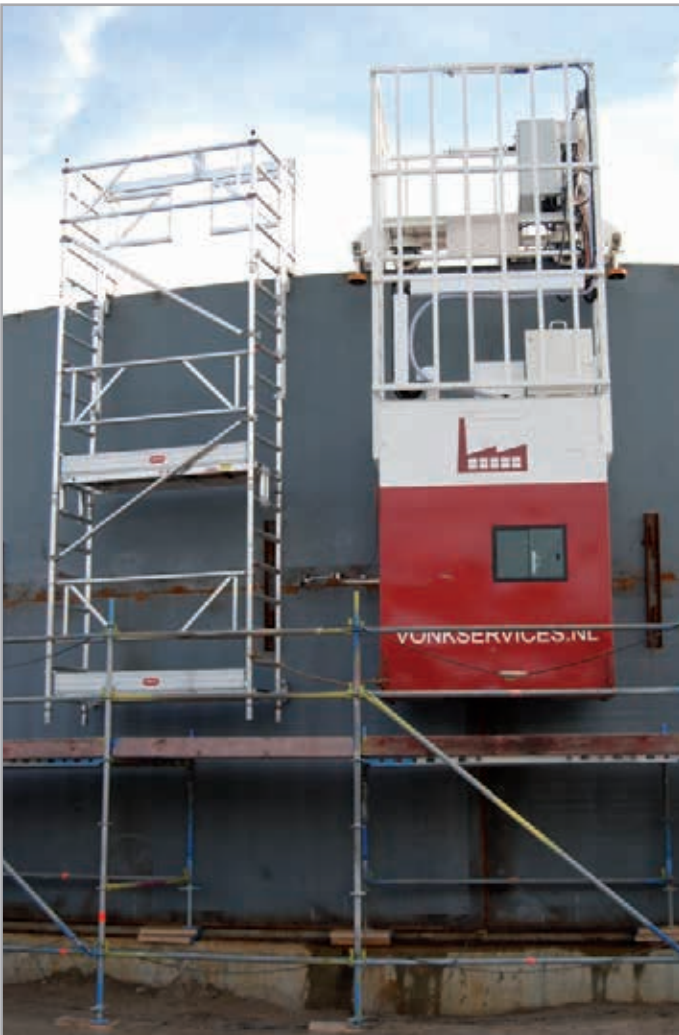
Welding scaffold for silos
