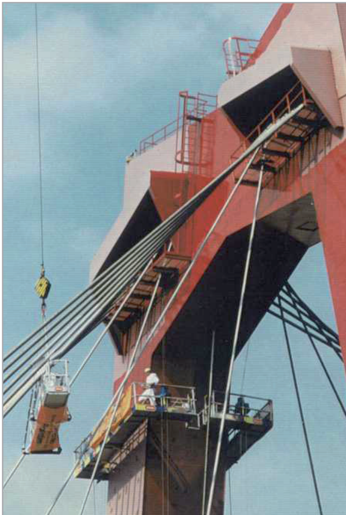
Maintenance platforms for a bridge
