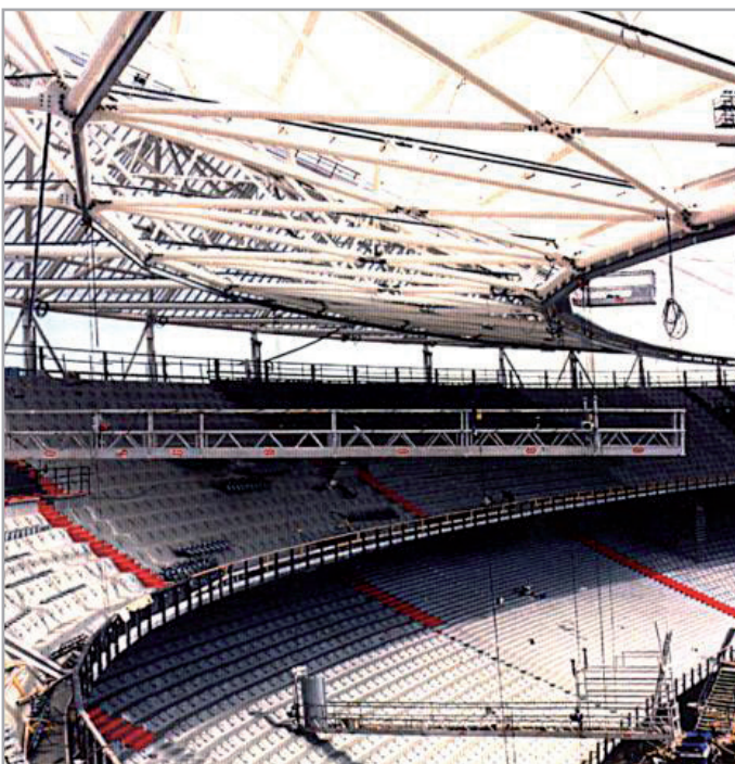
Maintenance platform Football Stadium
