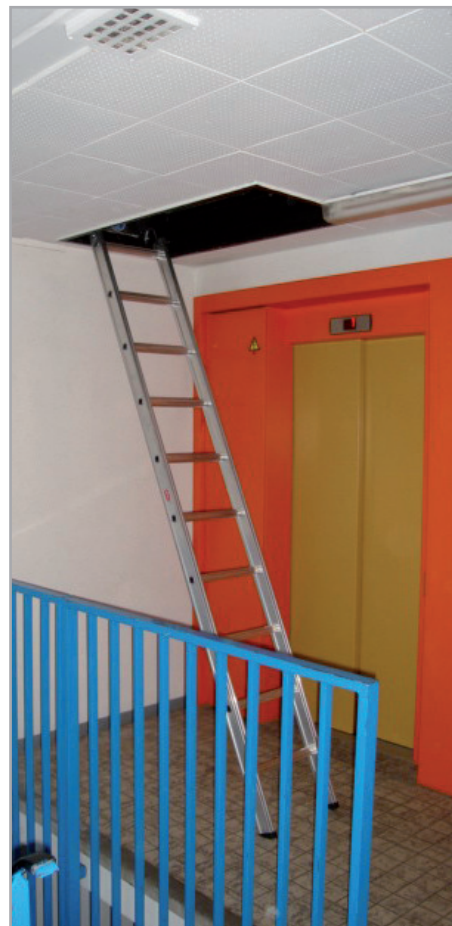
Custom-made ladder with hooks to provide access to the hatch
