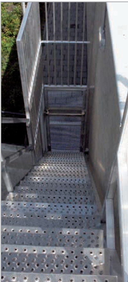
Escape route/fire escape stairs with perforated steps and anti-theft protection railing
