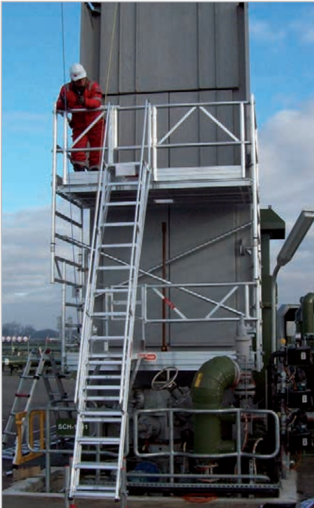
Suspended scaffolds with access stairs
