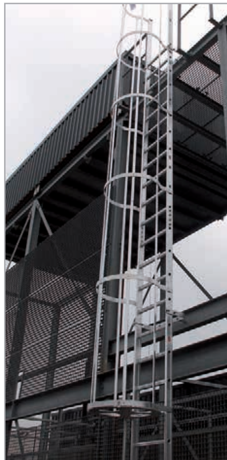
Hoop ladder with minimal anchoring
