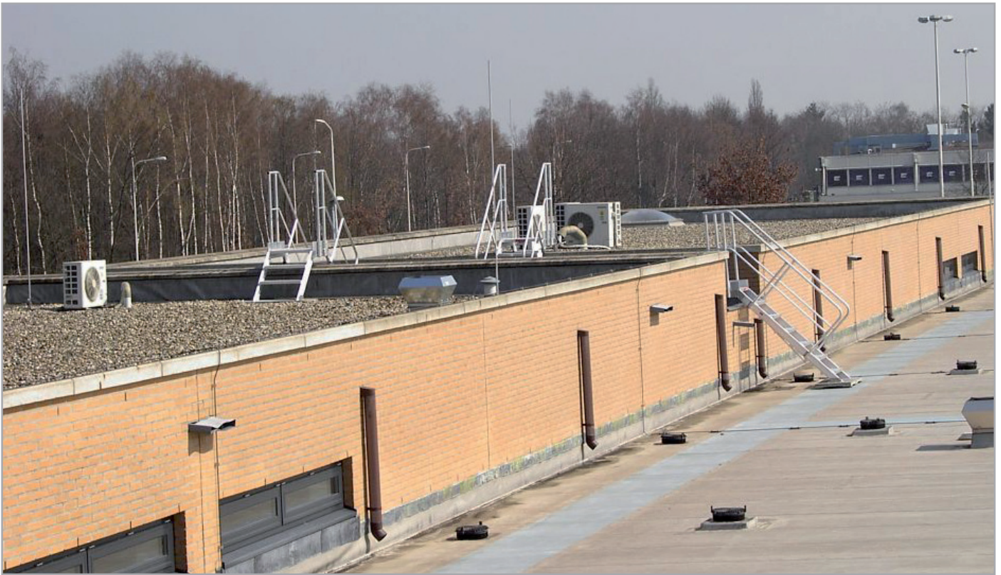
Step-over stairs and straight stairs for safe roof access
