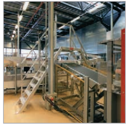
Industrial step-over/stairs in factory
