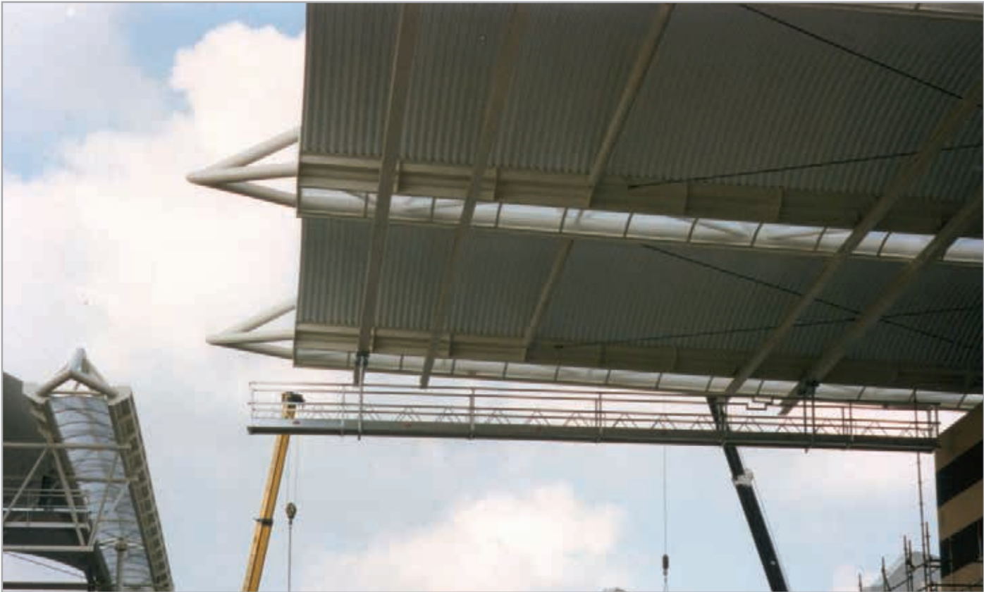
Maintenance platform Football Stadium
