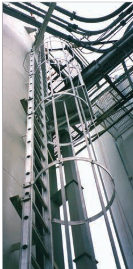
Hoop ladder with side step-off and step-off platform
