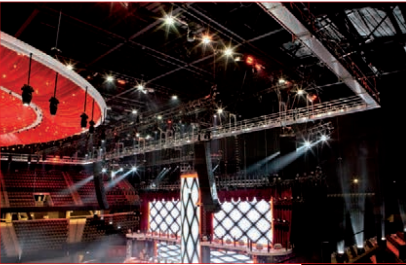
Suspended catwalk during Music concerts (240 meter long)
