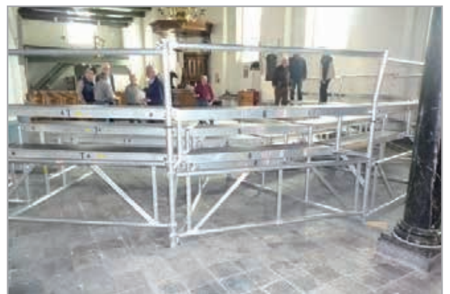
Podium made out of scaffolding components
