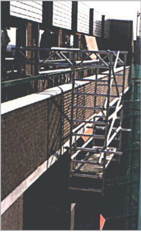
Suspended scaffold various working heights
