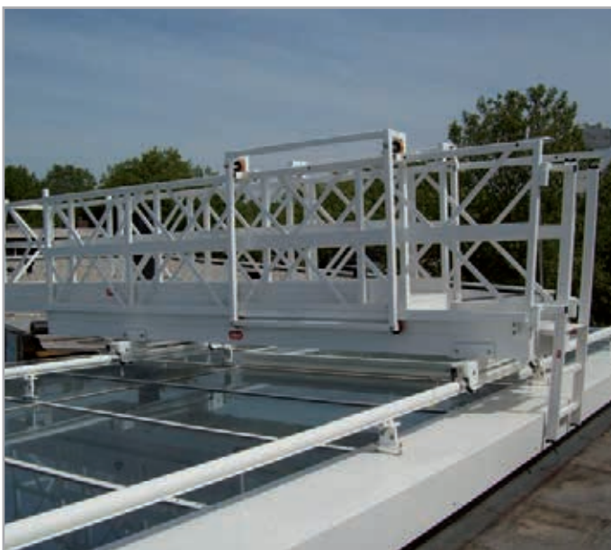
Mobile maintenance platform on glass roof
