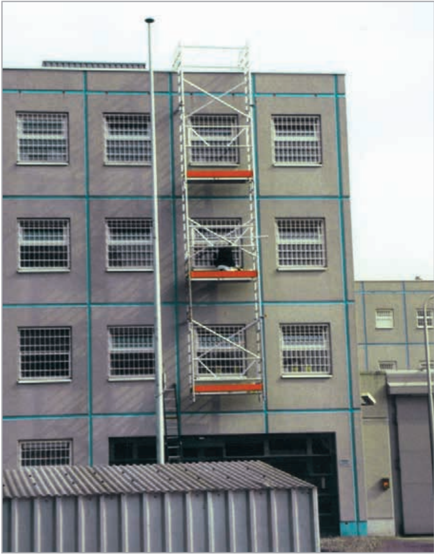
Suspended scaffold narrow
