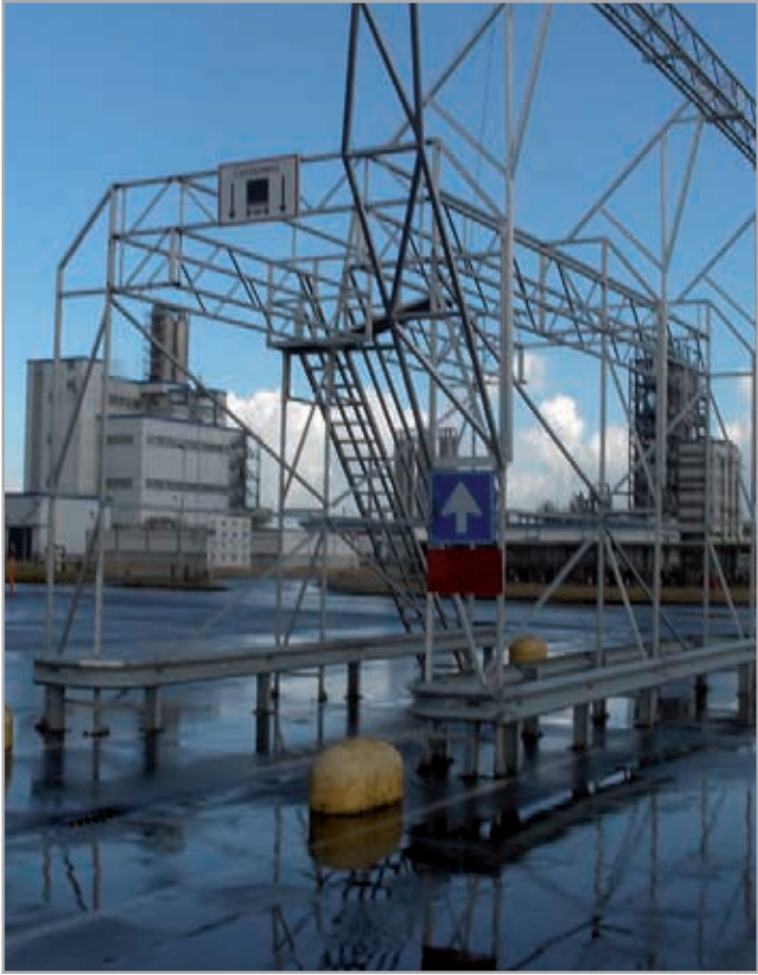
Load protection system for trucks
