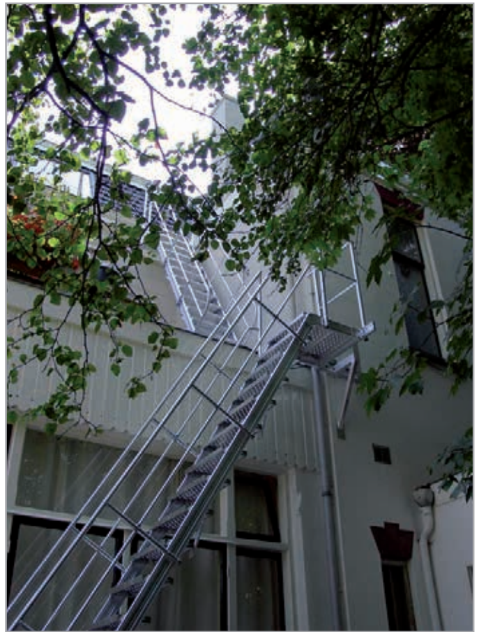
Aluminium straight ladder with rest platform for use as an escape route
