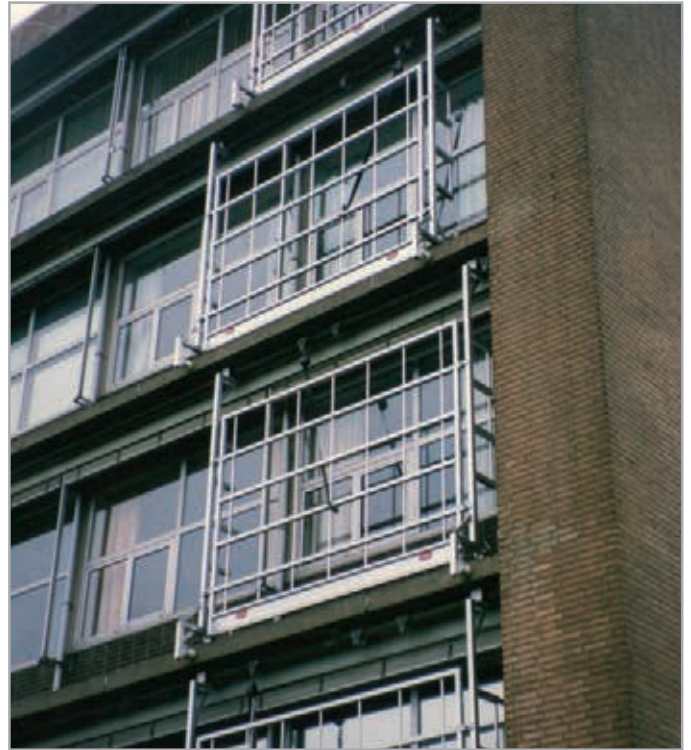
Fall protection for balconies
