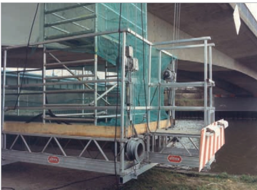
Suspended platform under the Zeeland bridge
