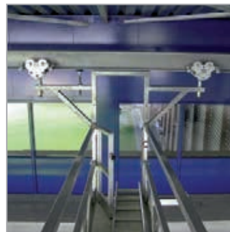
Rollable suspension frame maintenance platform
