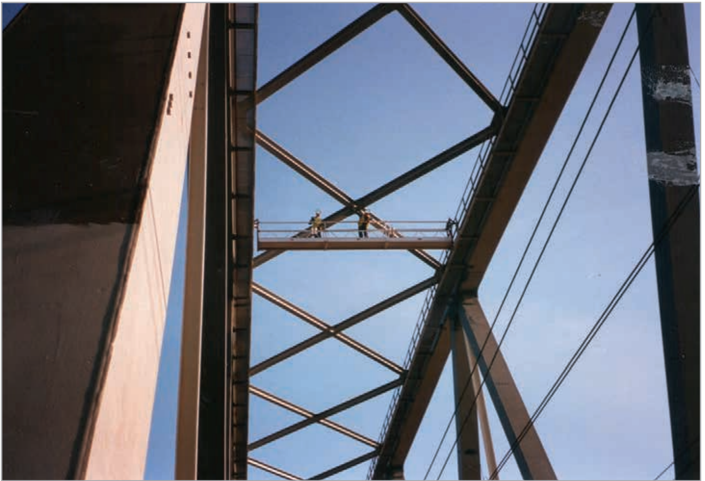
Working platform (at the bridge over the river Waal Nijmegen)
