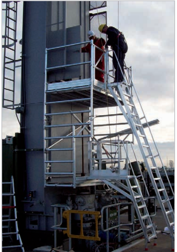
Suspended scaffolds with 2 working heights and access ladders
