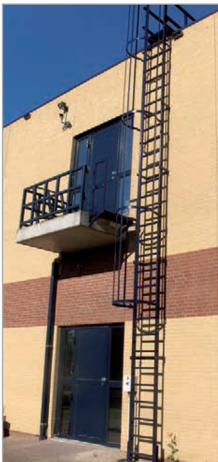
Coated hoop ladder with step-off platform and side step-off
