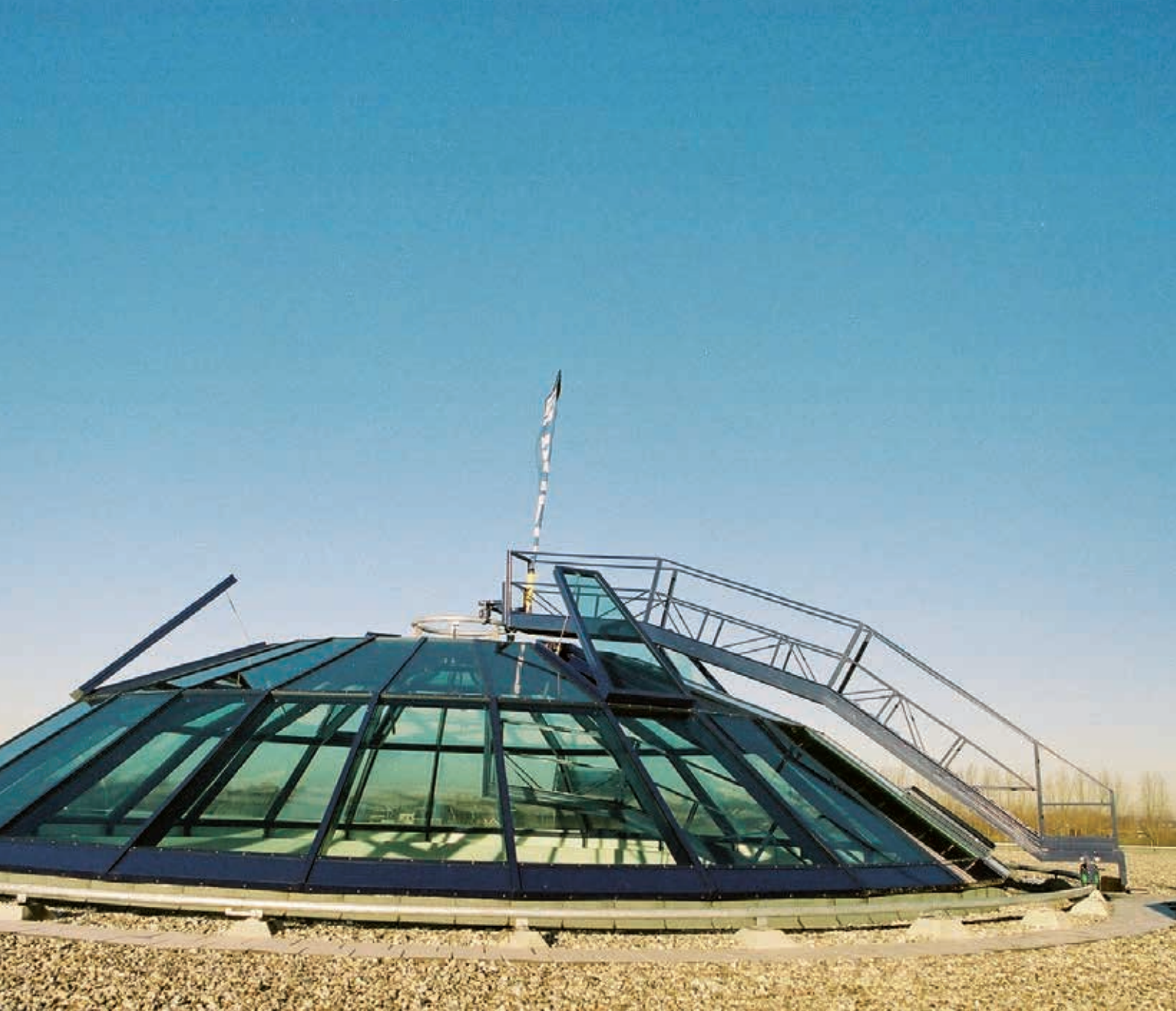
Permanent access gantry on roof
