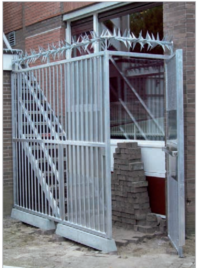
Fire escape stairs with railing with rotating point protection
