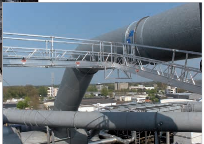
Walkway between pipelines
