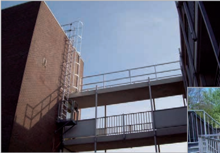
Hoop ladder with railing
