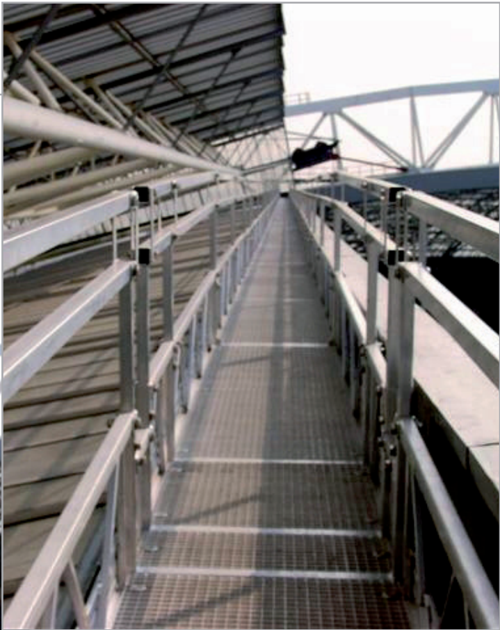
Maintenance platform Football Stadium
