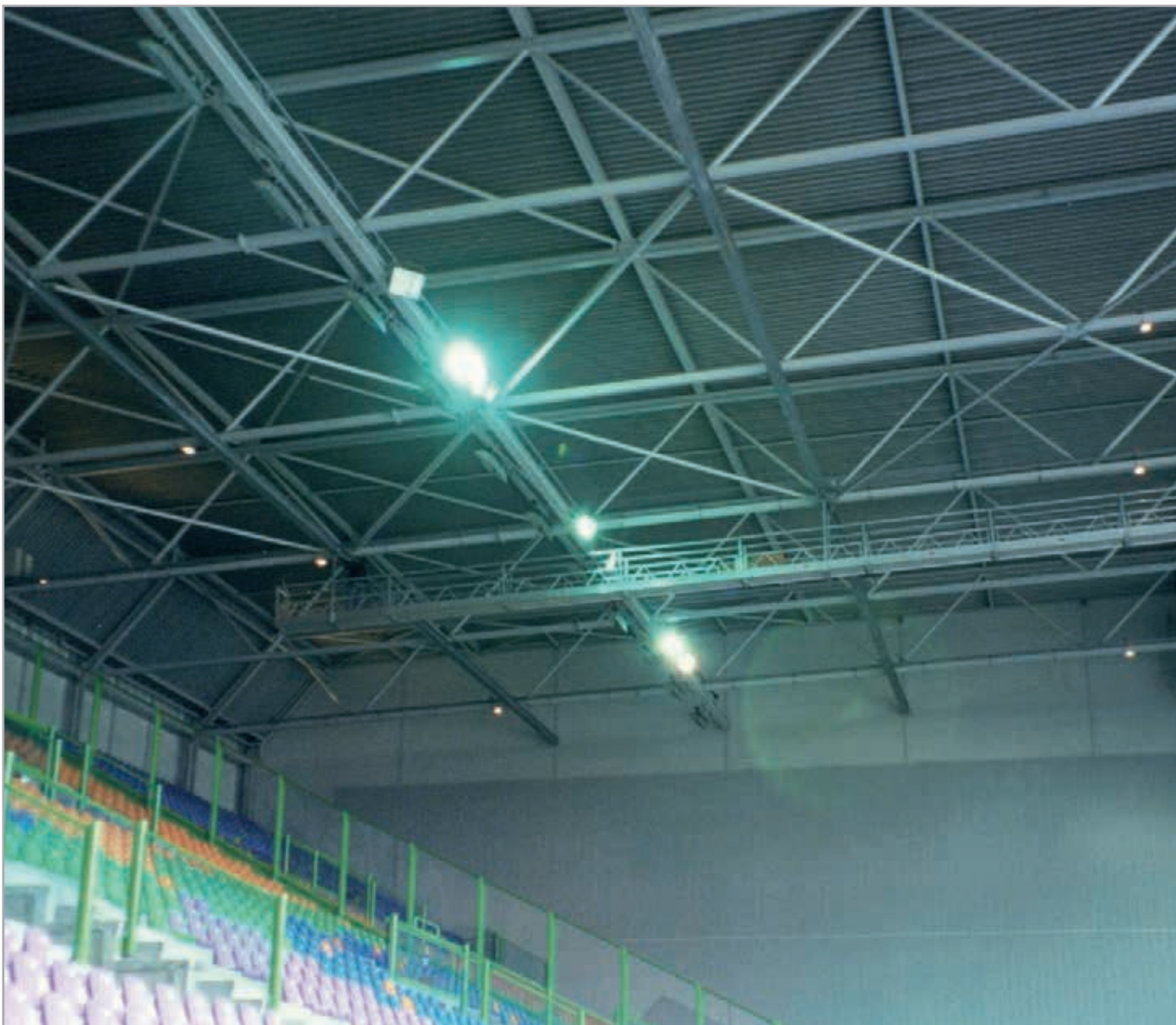
Maintenance platform Football Stadium
