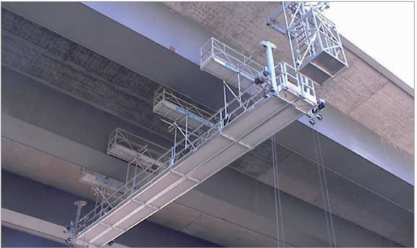
Working platform under a bridge
