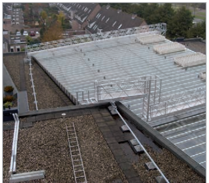
Mobile working platform over glass roof
