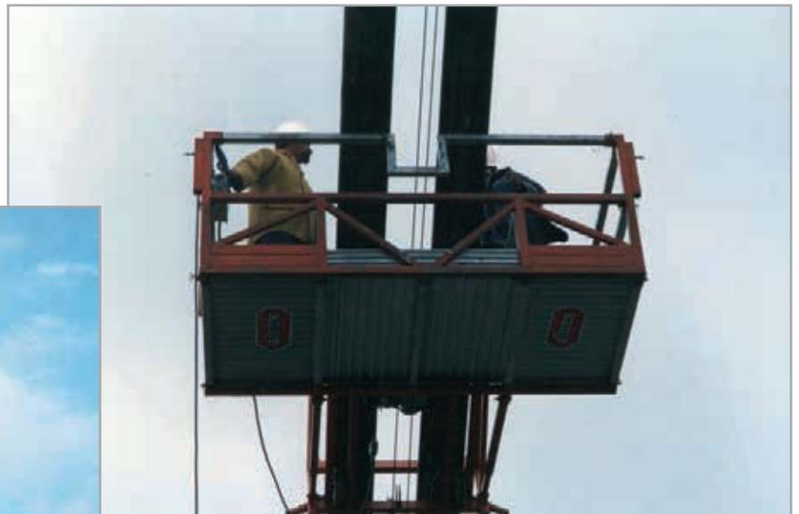
Mobile working platform on the suspension cable of a bridge
