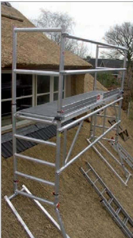
Dormer window scaffold for a straw roof
