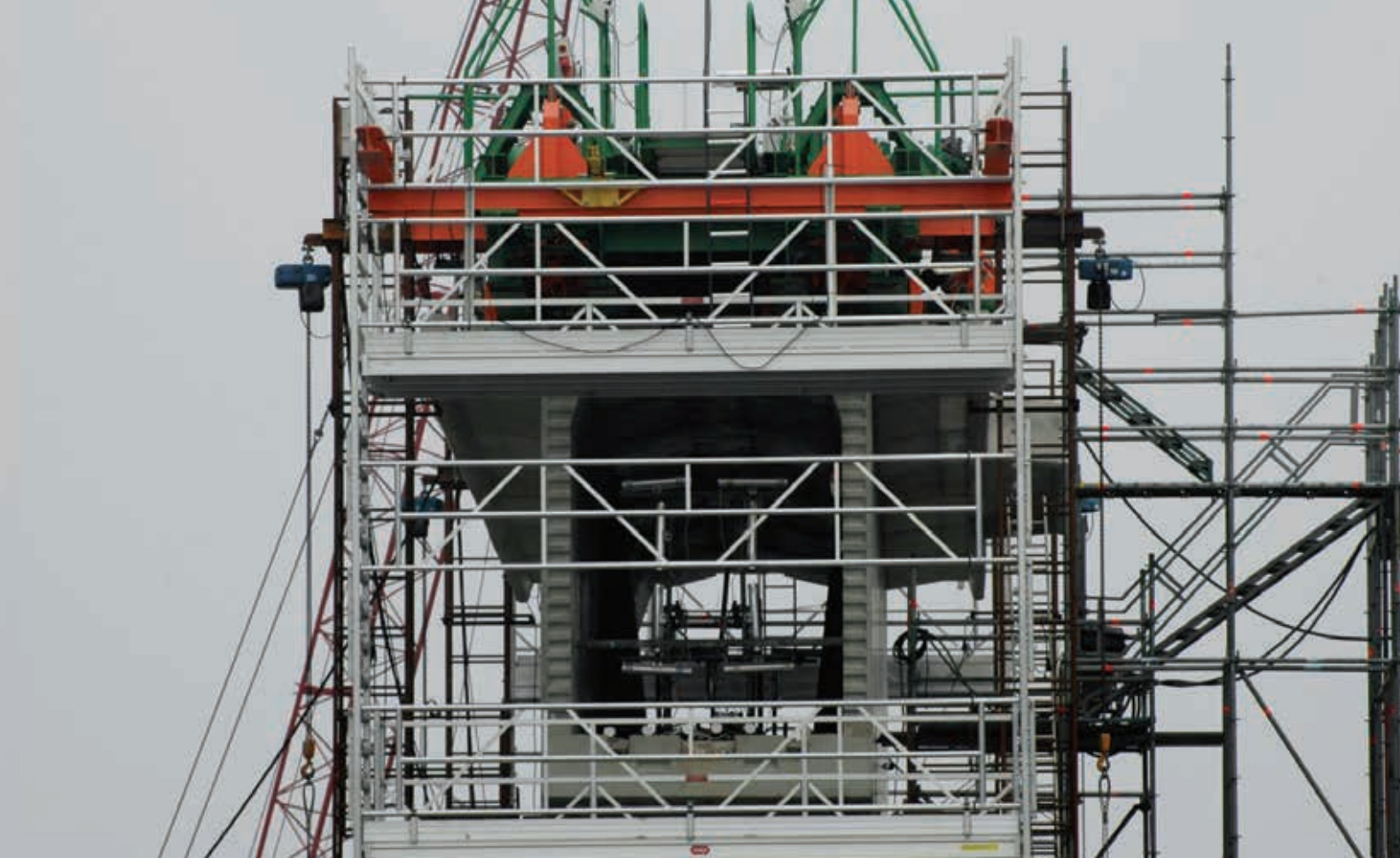
Suspended scaffold under a bridge
