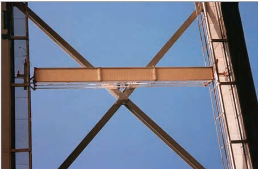
Painters platform (at the bridge over the river Waal Nijmegen)
