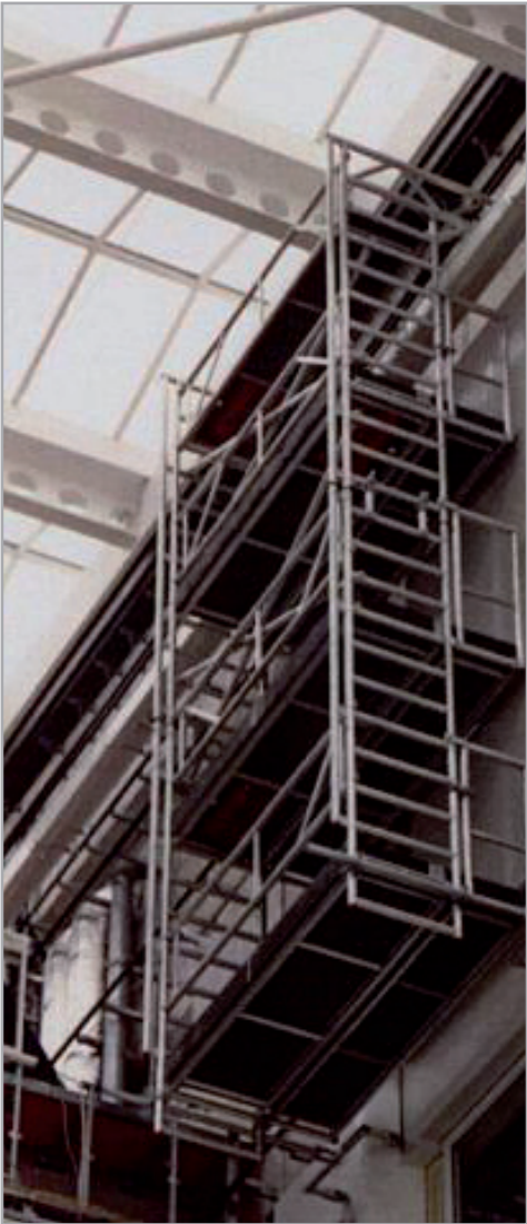
Suspended scaffold with 3 work levels
