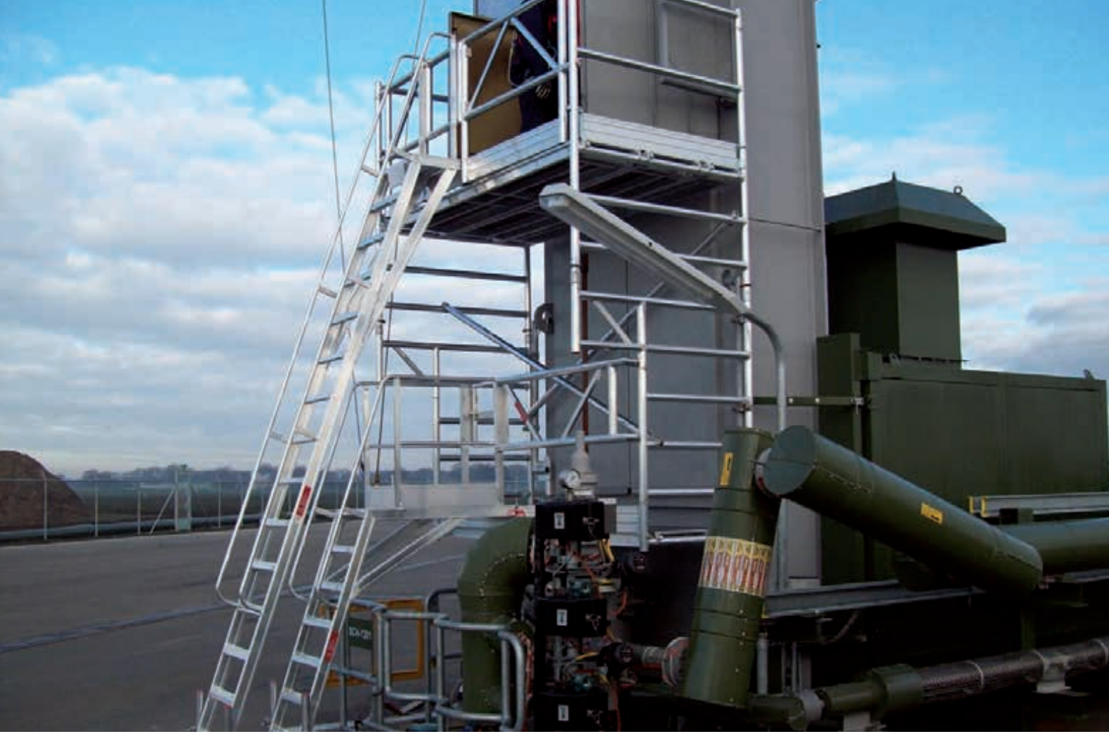
Suspended scaffold with access stairs (NAM)
