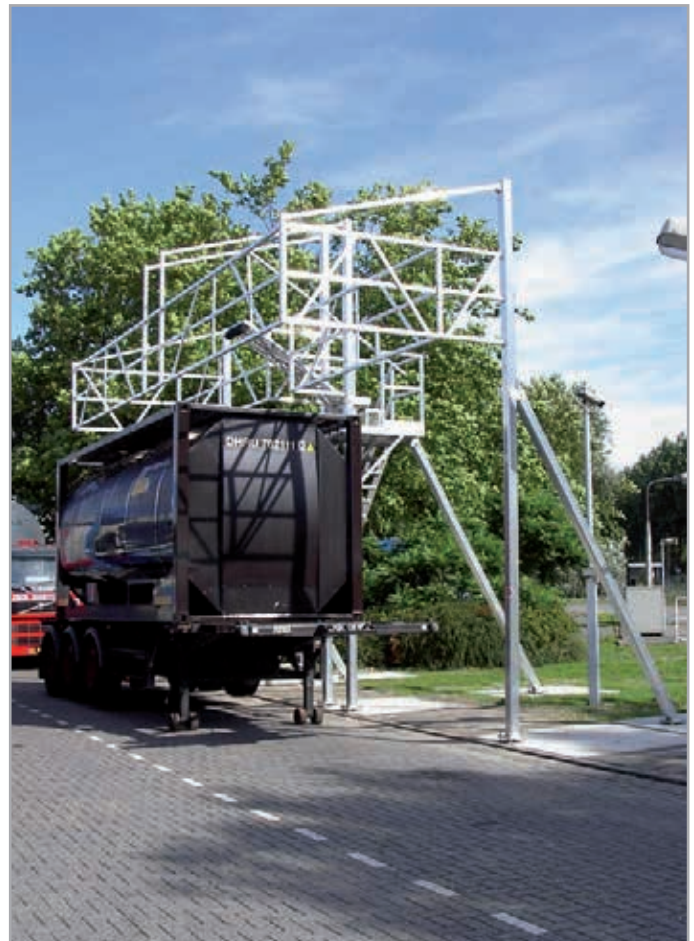
Fall protection system for tanker trailers
