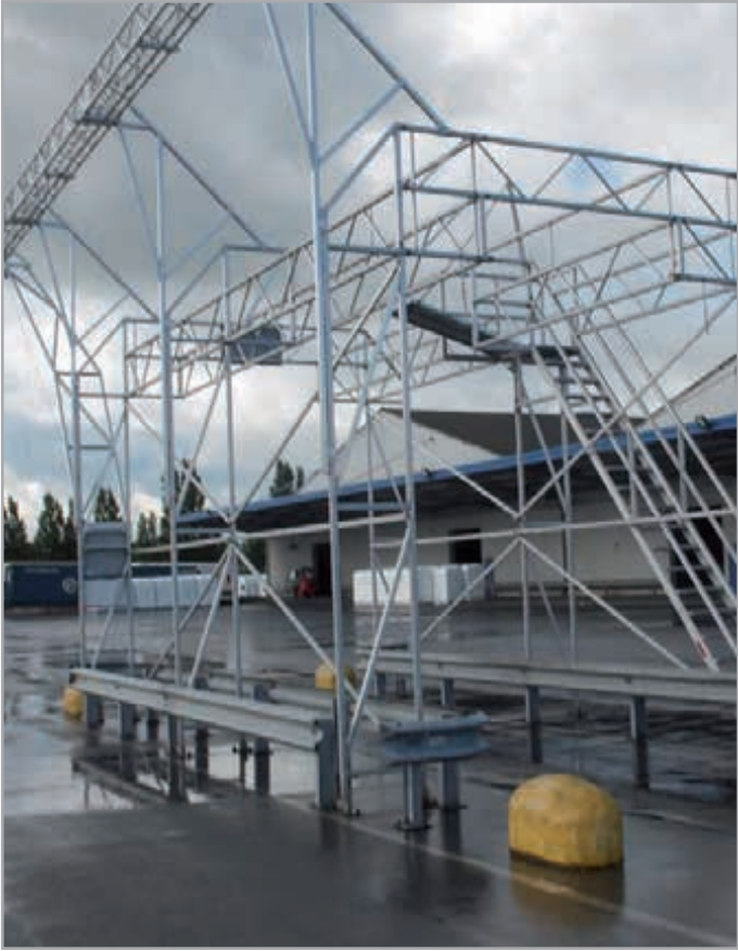
Fall protection system for trucks' loads
