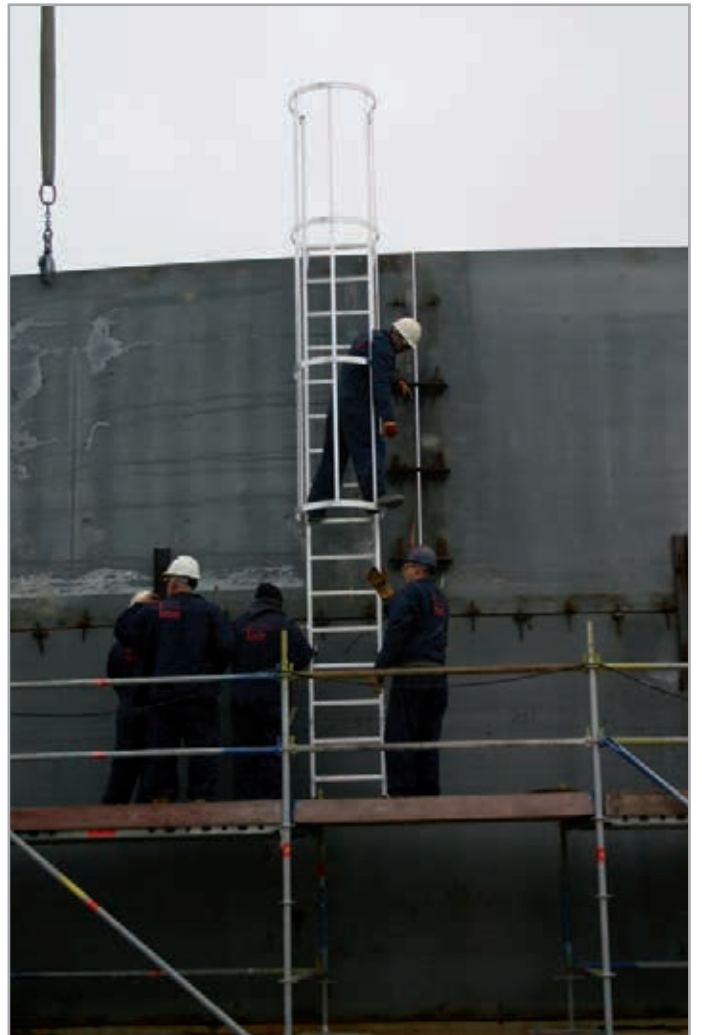
Mobile hoop ladder on roof of a silo
