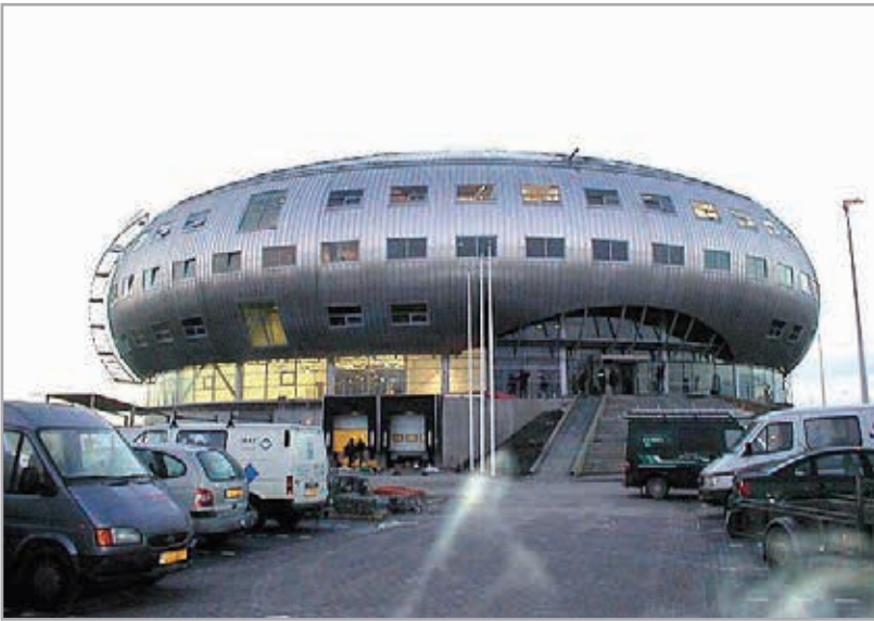
Window cleaning working platforms façade maintenance
