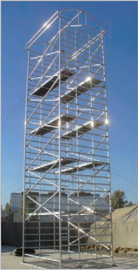
Special scaffold for parachute drying tower Air Force Defence
