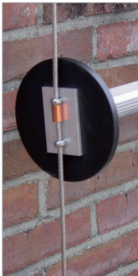
Steel cable ladder rung connection
