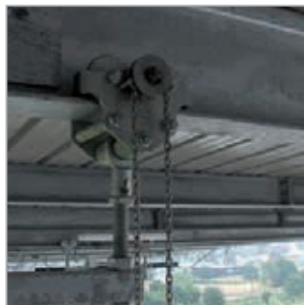
Sideways movable suspension frame maintenance platform
