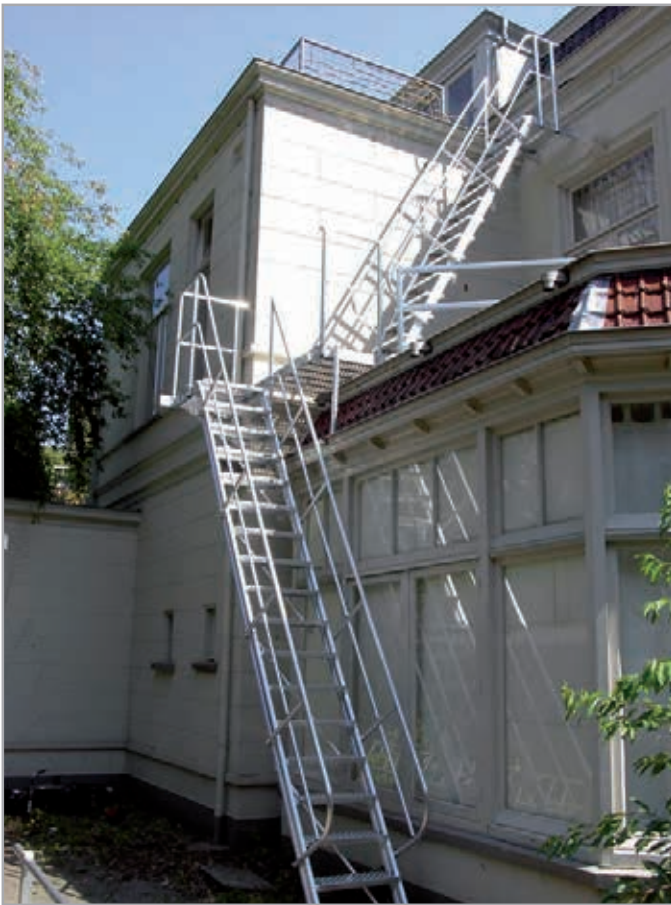
Escape route/fire escape stairs with in between platform
