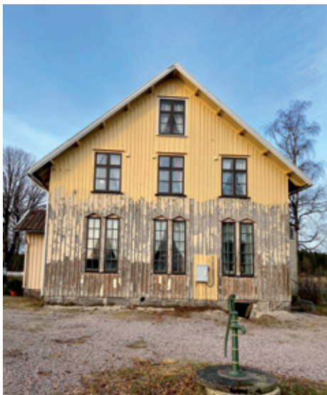
Nothing is too difficult for Allbäck Linseed Oil Paint. Scrape to a solid surface, clean, stain and finish painting.
