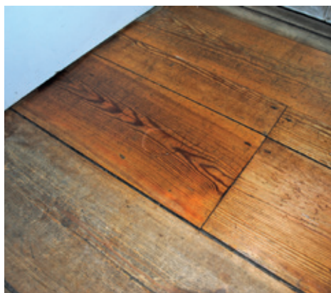
Linseed Oil Wax Natural used on old wood. Before/after treatment.
