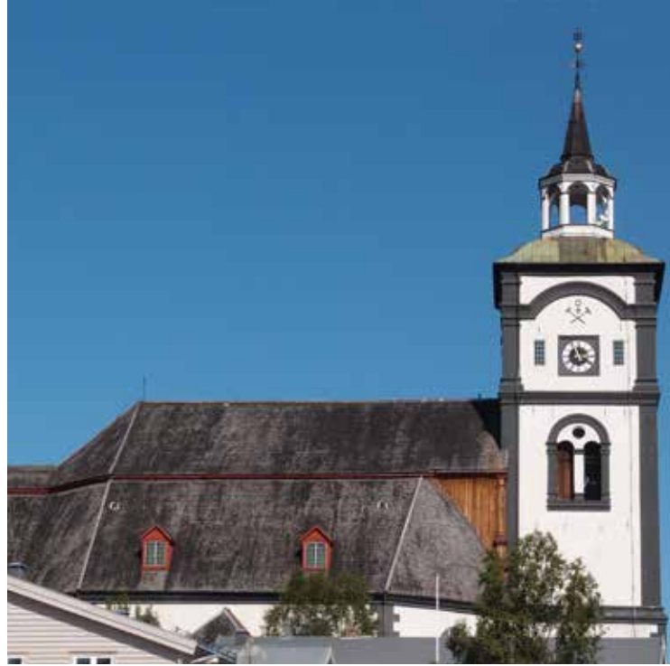
Stav chips with "armor" layer of tar, coal and sand on the Roros church in Norway, is from the 1700s. Photo: Sara Höglund.
