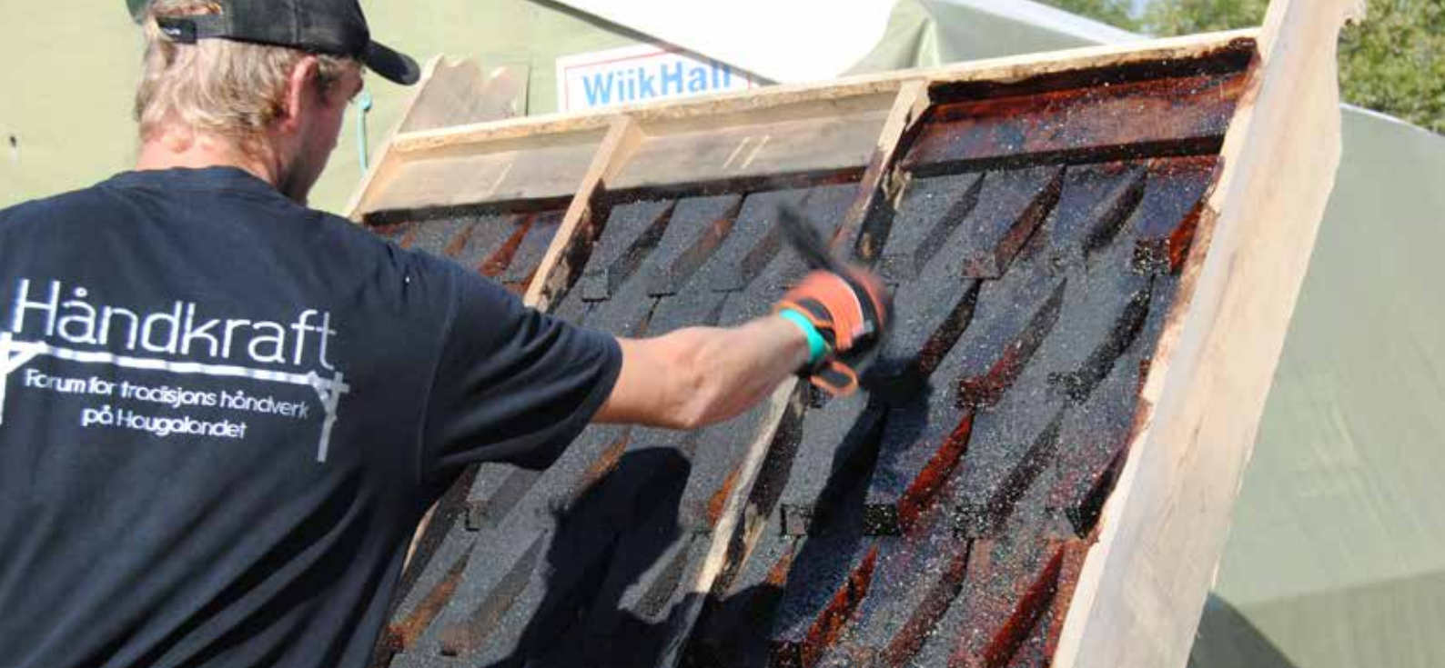
during bygningsvernkongressen in Oslo in 2014 was made craft experiments with sand on tarred rod turnings. Photo: Christina Persson.
