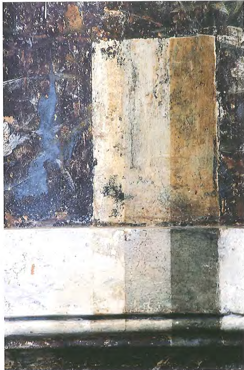
A paint survey on site enables previous paint treatments to be uncovered and determined. In most cases, a paint survey plus an archive search provides sufficient information to reconstruct a previous paint treatment.
