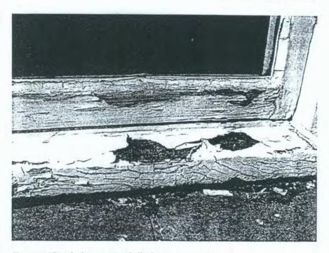
Figure 2 Detail of conventional alkyd paint on a Holkham estate cottage six years after it was painted, showing paint cracking, flaking, and allowing water ingress leading to timber decay. Note that the paint has also flaked off the putty, which itself has hardened and cracked, requiring replacement.
