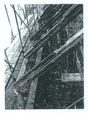
Figure 4 The rafters of the Fig House in the Holkham kitchen gardens. The 1872 timbers have benefited from the application of warm raw linseed oil. Note the lightness of the as-yet-untreated timbers and the relative lack of new wood required in these repairs, undertaken during 2001.
