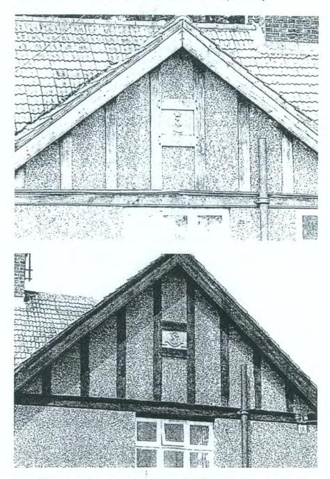
Figure 6 The oak timbers on these buildings show the rejuvenating effect (before and after) that a coat of warmed, raw linseed oil can have.
