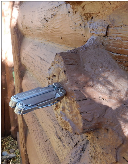
Fig. 3. Only a shell of waterborne paint is holding these decayed, hollowed-out log crowns together after decades of repainting with new waterborne latex and acrylic paint. Regular repainting without examining the condition of the underlying wood resulted in built-up paint layers that hid the wood decay, 2016.
