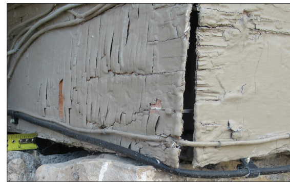
Fig. 5. Many painting campaigns have led to overpainting and a film thickness of around 1 millimeter in areas on this wood sill trim board, 2020.
