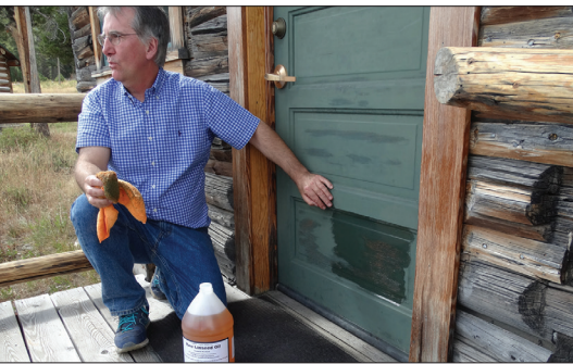
Fig. 6. A south-facing door at White Grass Ranch that was painted with linseed-oil paint has chalked after four years and is here being rubbed with purified linseed oil to refresh the paint film. Doors facing to the east, west, and north required re-oiling after eight years, 2016.
