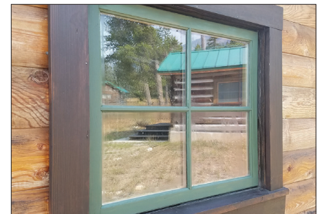
Fig. 7. Window at White Grass Ranch before the introduction of linseed-oil paint when waterborne latex paints were used, 2020. This window had early signs of paint failure, such as cracking and peeling, after two years. After 10 years, the paint had flaked off the bottom rail, portions of both stiles, and three muntins. This condition caused window glazing to fail in areas and required scraping and removal of loose paint, partial reglazing, and refinishing.
