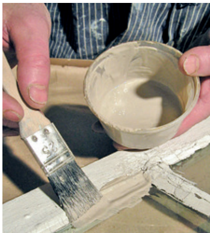
Thinned putty – an easy "anti-aging" measure.
