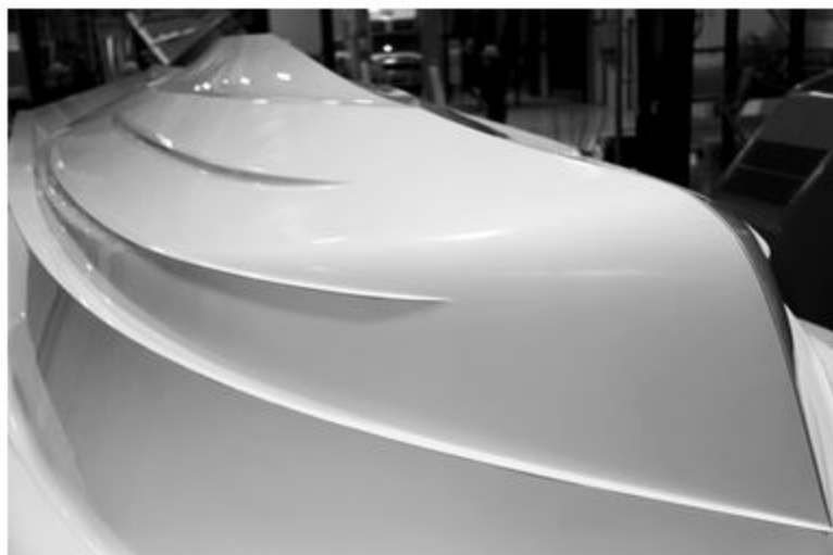
The Icelandic Coast Guard's Leiftur under construction
