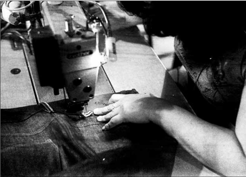
**Fig 9** Sewing the leather tab on to each pair of jeans is one of many processes requiring specialized equipment. Photograph by Nick Pironio.
