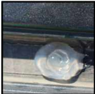
Next apply silicone over the holes
