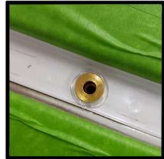
Insert into the roof.
