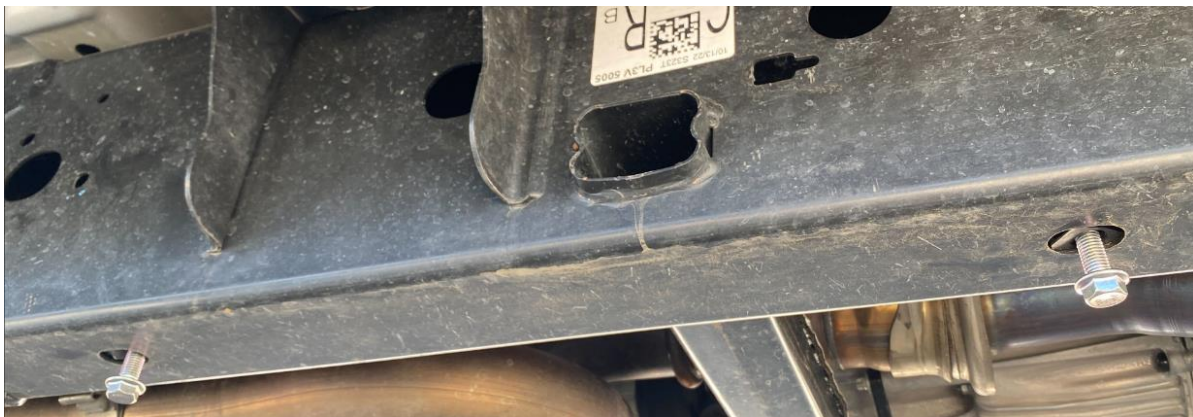
Figure 16: Preinstallation of Lower M10 Bolt
