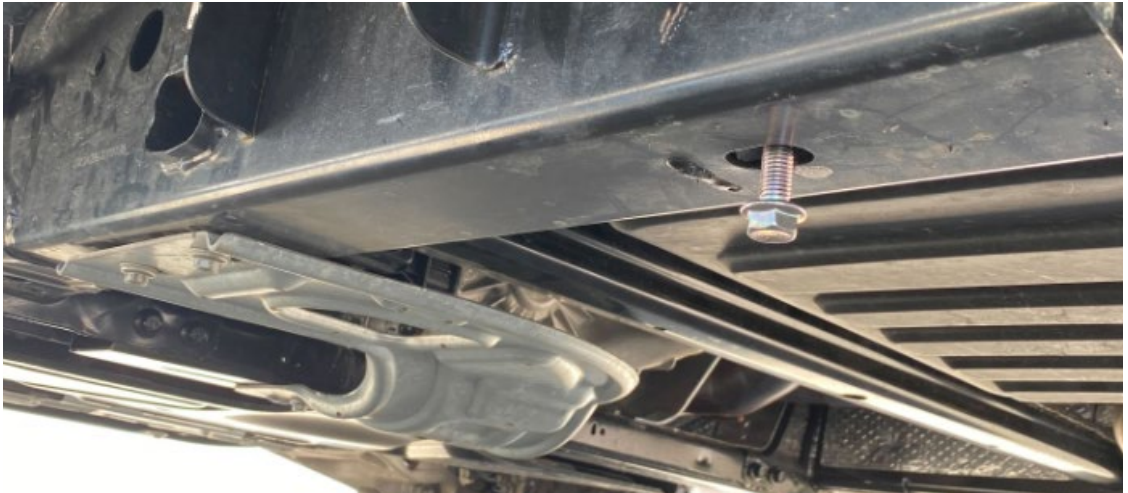
Figure 8: Preinstallation of lower M10 bolt
