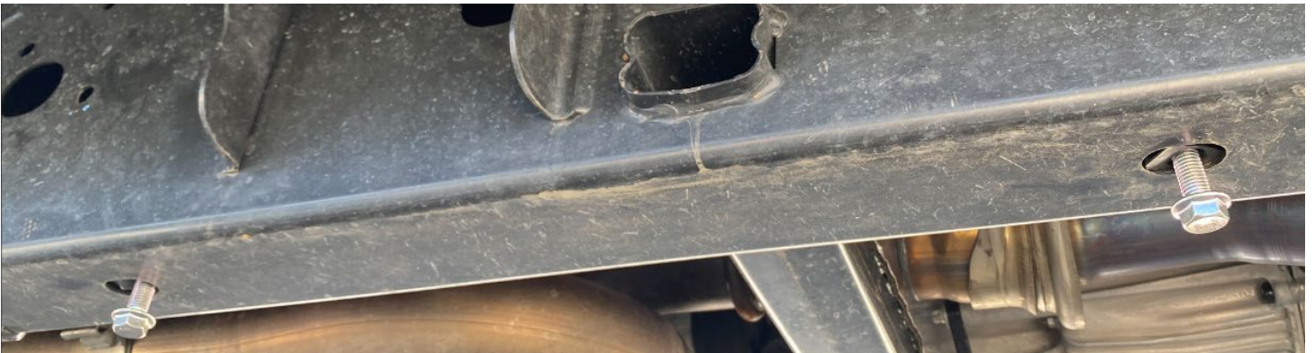
Figure 18: Preinstallation of Lower M10 Bolt
