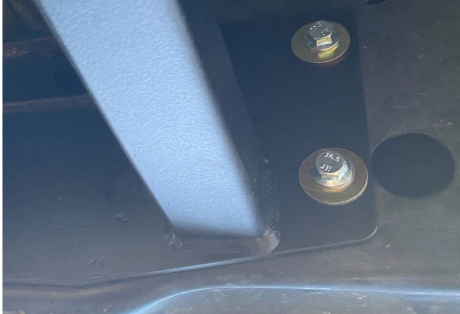
Figure 13: Correct installation of M10 bolts
