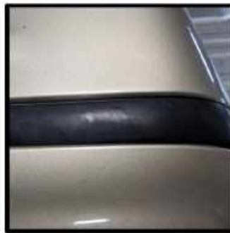
Locate and remove the gutter trim on the roof
