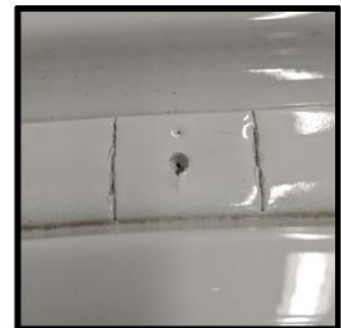
Repeat on the otherside, these will be the locations of the first mounting holes
