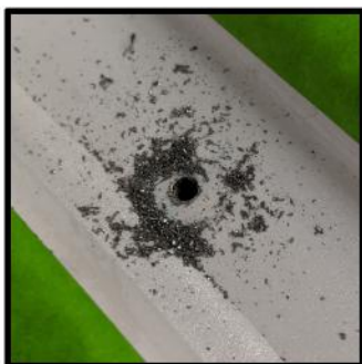
Remove the factory channel sealant and drill pilot holes
