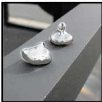
Apply a generous amount of silicon to the holes as shown above
