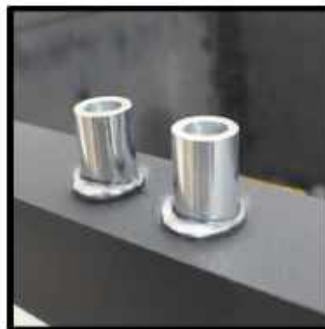
Next place the spacers on the roof
